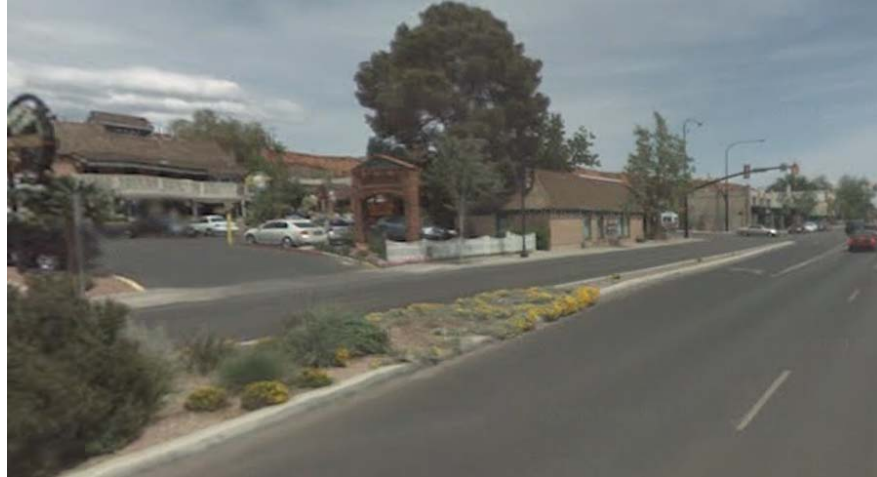
Figure 3-5. Raised median on St. George Boulevard (SR 34) (Google 2010).
