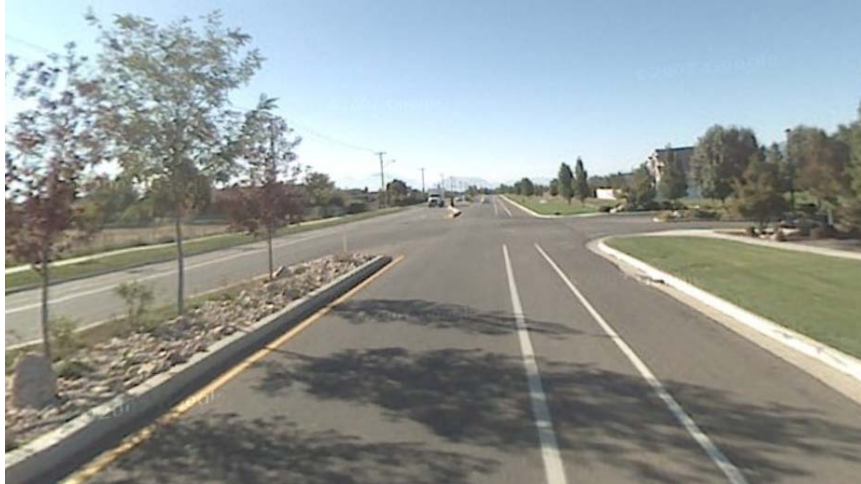
Figure 3-2. Raised median on Alpine Highway (SR 74) (Google 2010).
