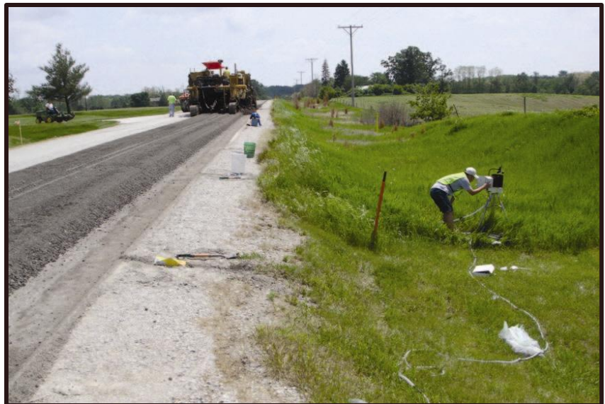
Installation of weather station
