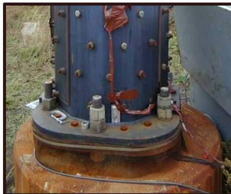
Bolted Reinforcing Jacket
