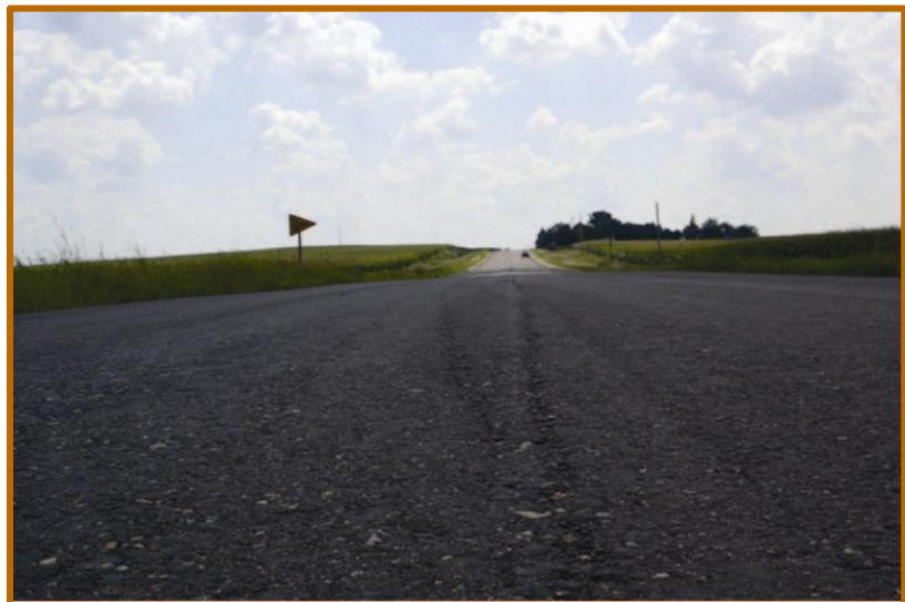
Curing process on Iowa county road before overlay
