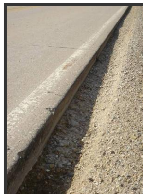
An example of granular shoulder edge rutting Photo: Dr. David White, Iowa State University/InTrans
