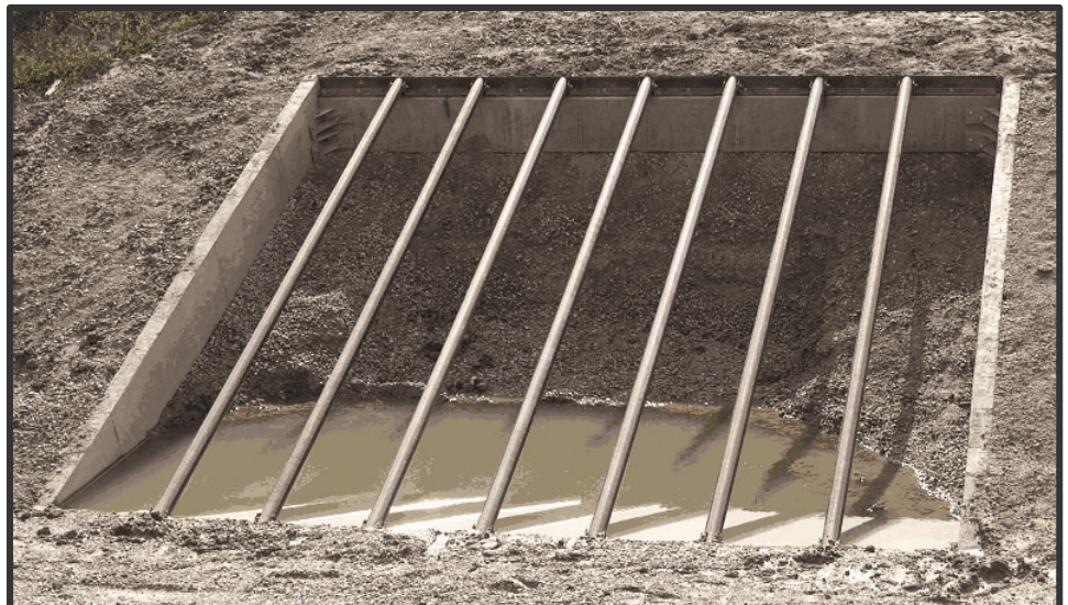
Safety treatment for cross-section drainage culverts
