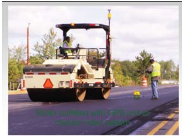
Roller coverage as determined by GPS Data
