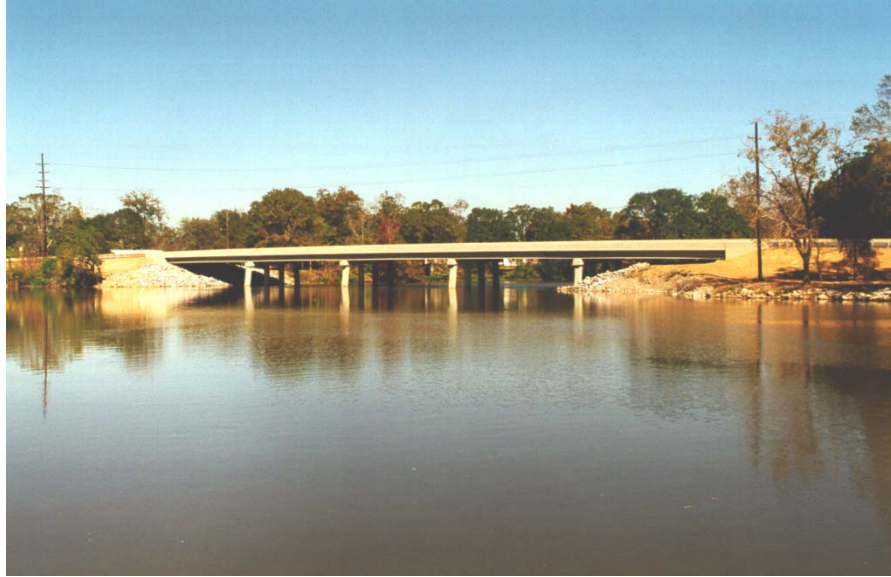
Figure 2 New Charenton Canal Bridge
