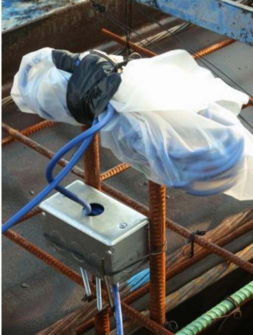
Figure 49 Protection of wiring for embedded sensors prior to concrete casting
