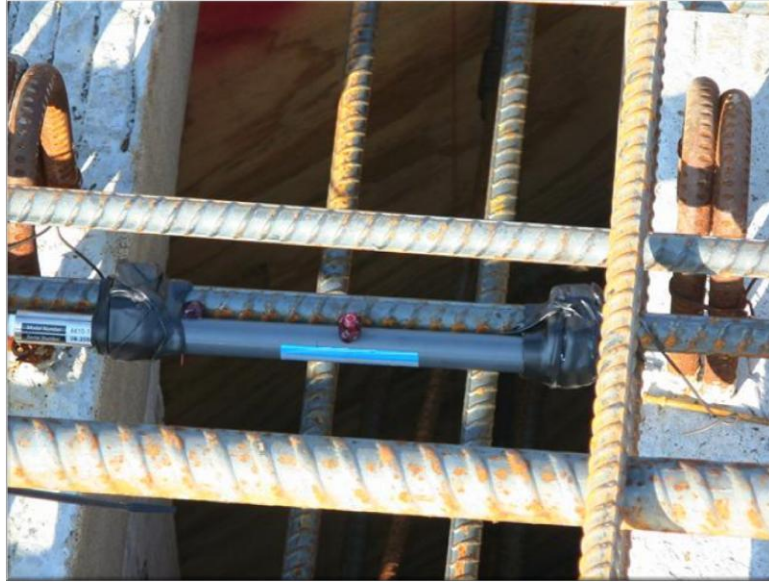
Figure 45 Strandmeters installed on reinforcing bars in deck over continuity diaphragm
