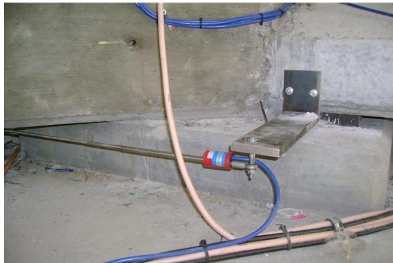
Figure 48 Gap meter installed on brackets connected to girder ends at continuity diaphragm
