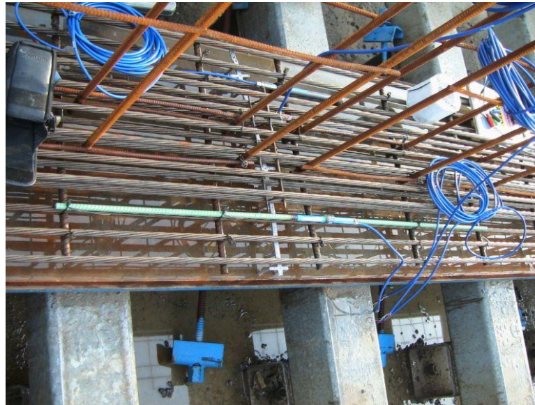
Figure 44 Sisterbar installed next to a prestressing strand at midspan
