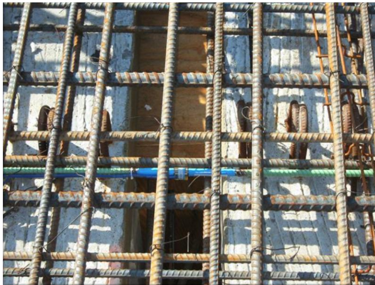
Figure 46 Sisterbars installed next to reinforcing bars in deck over continuity diaphragm
