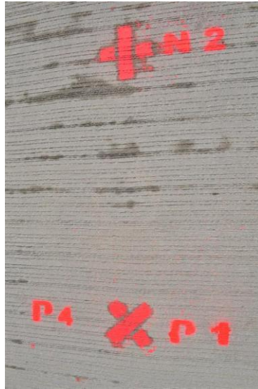
Figure 23 Marking the bridge deck at truck positions for static live load test
