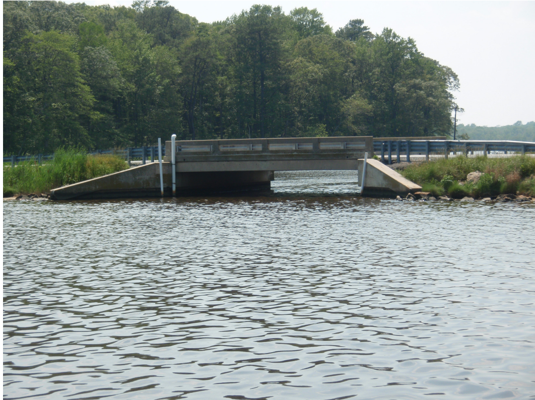
Figure 5.10 Picture of Old Mill Bridge looking north (Photo: Hayes 2008).
