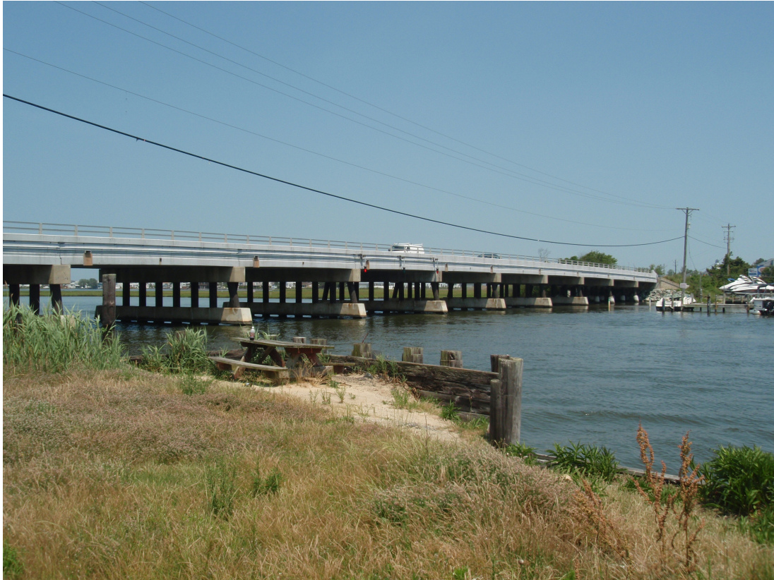
Figure 5.6 Picture of Fenwick Island Bridge looking north (Photo: Hayes 2008).
