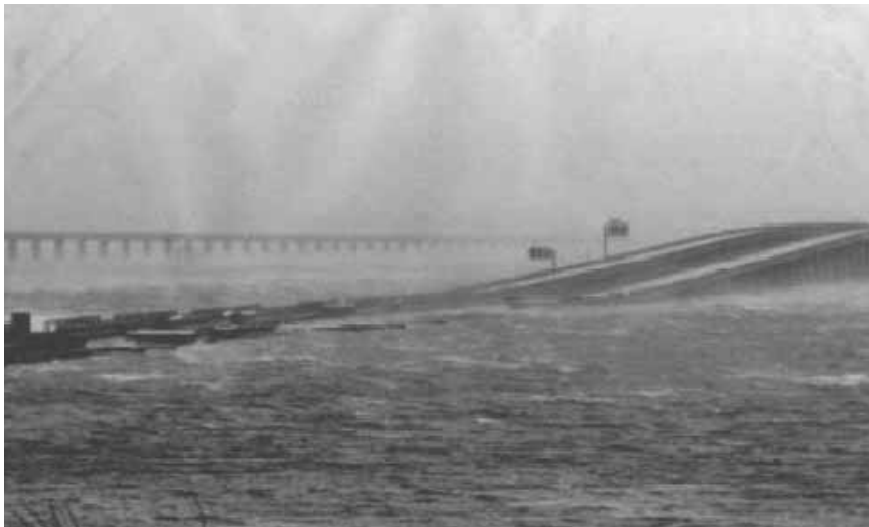
Figure 2.1 I-10 Bridge over Escambia Bay during Hurricane Ivan (Sheppard).
