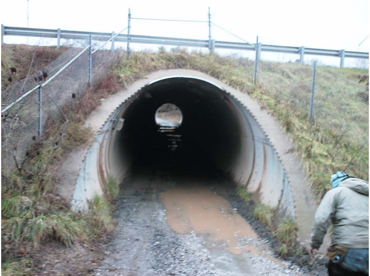
Figure 3. Culvert 02159X0 functions as an equestrian underpass. It is 15 feet (4.5 m) in diameter, 242 feet (73.7 m) long, and essentially dry. This cylinder culvert cell has 5 feet, 10 inches (1.8 m) of type 1 fencing and a gravel substrate.
