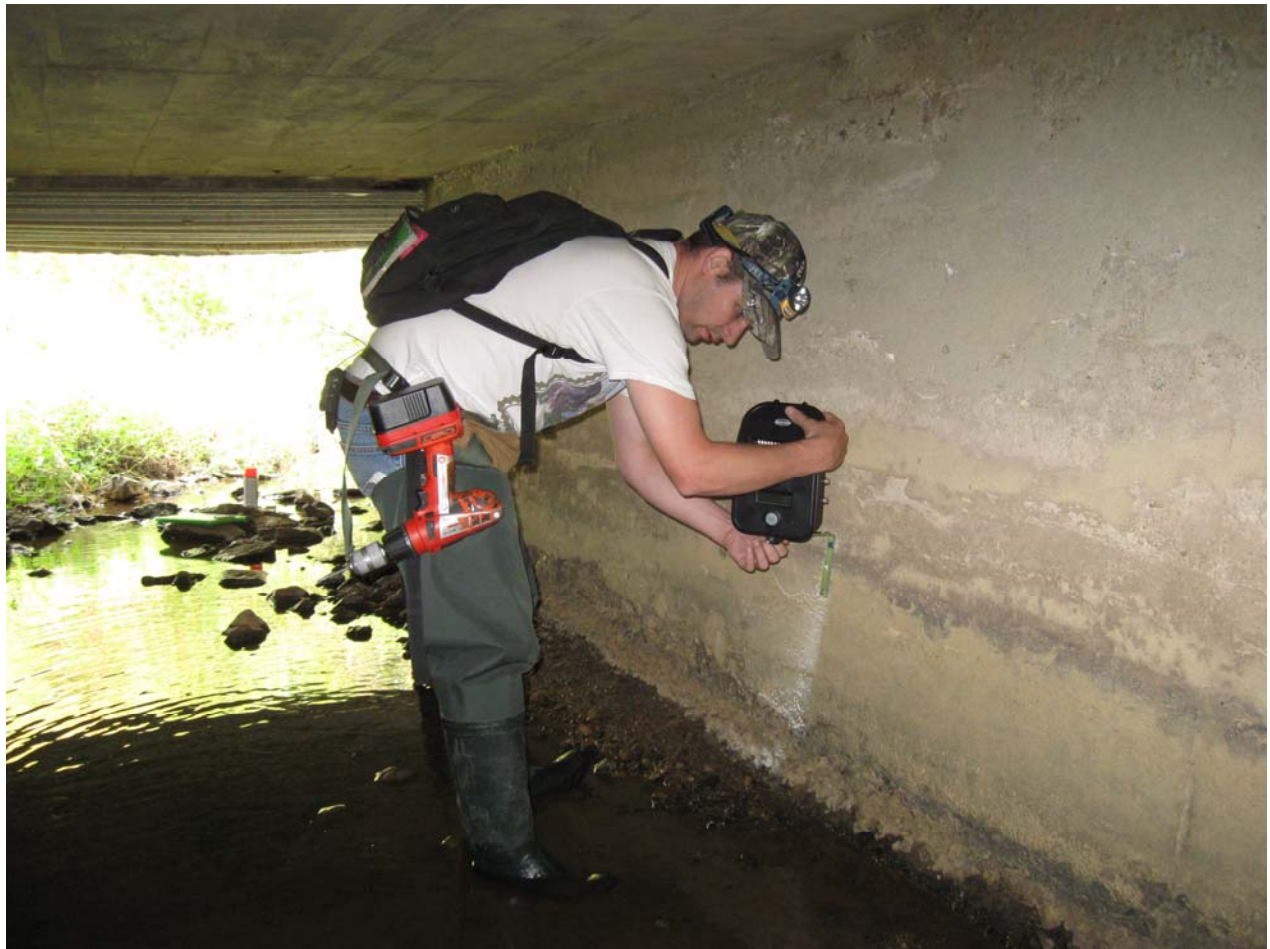
Figure 4. Installation of an infrared, motion-detecting trail camera on an angle bracket in a box culvert.
