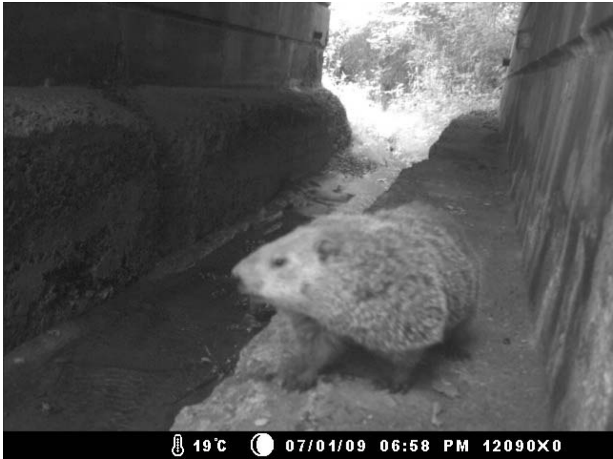
Figure 9. A woodchuck is caught using an existing ledge in a box culvert.
