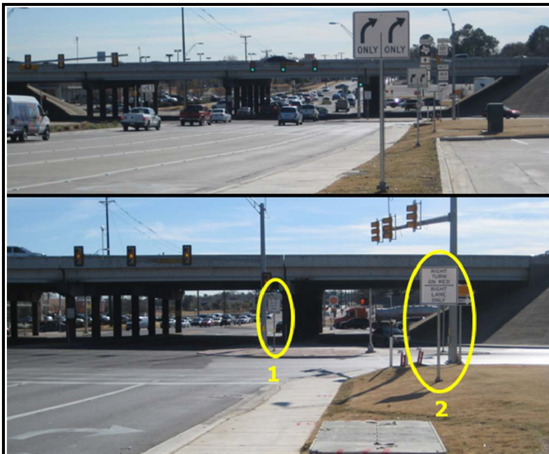
Figure 7-9. Precinct Line at SH 183 Dual Right-Turn Lane Signs and Markings.
