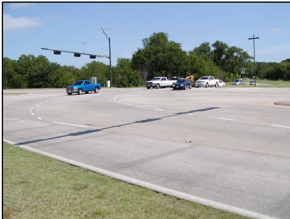
Figure 4-4. Pavement Markings at FM 2499 at Gerault Road Intersection.
