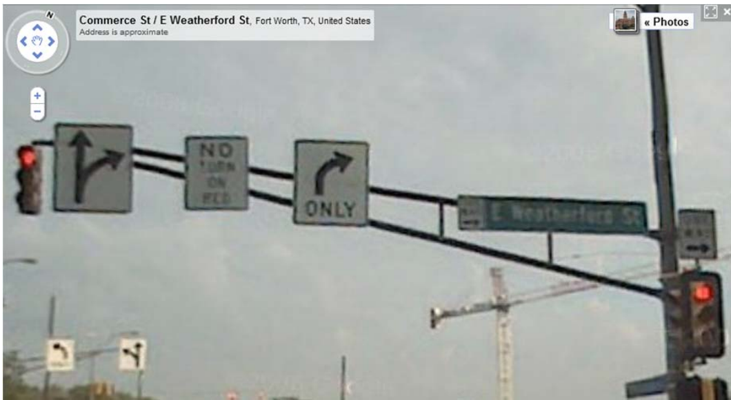
Figure 7-2. Advance Overhead Sign for Dual Right-Turn Lane.
