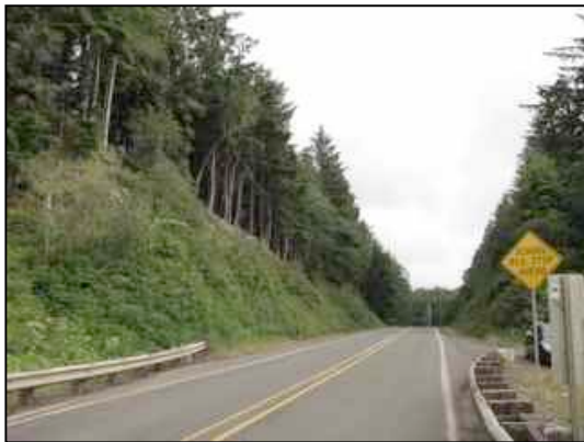
Figure 20. Roadway looking south
