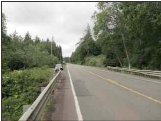
Figure 12. Rte 101 looking North
