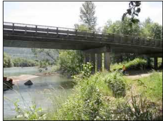
Figure 54. Looking towards inlet
