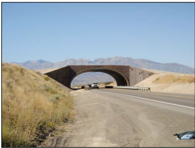
Figure 35. Example of a Class 5 Wildlife Overpass, NV © L. Bellis, Nevada DOT
