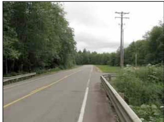
Figure 13. Rte 101 looking South
