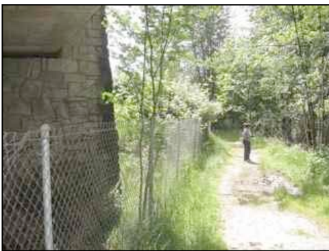
Figure 116. Chain link fencing
