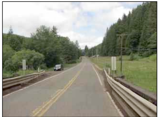
Figure 42. Highway 6 looking west
