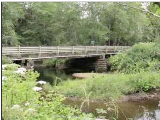
Figure 14. Bridge at Location 101_38.8_02
