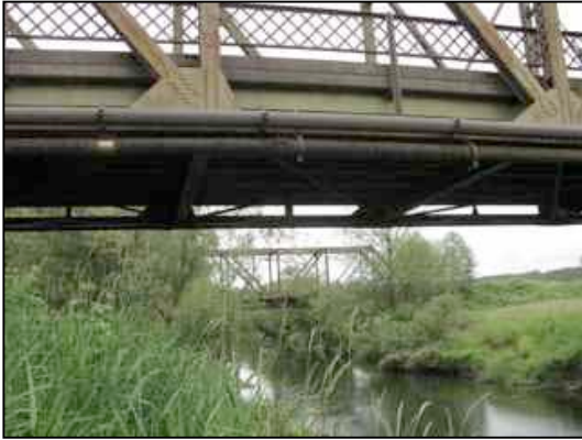
Figure 29. West looking towards bike path bridge
