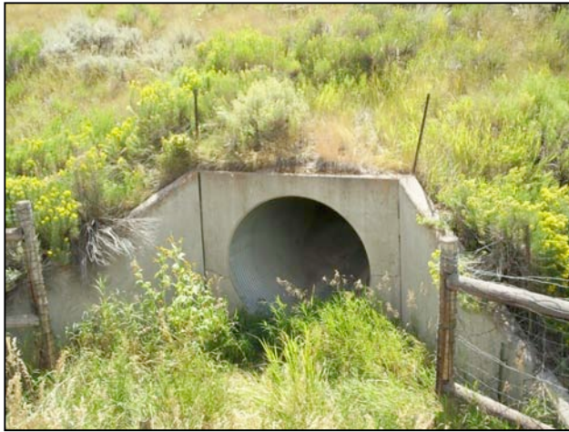
Figure 29. Example of a Class 1 Small Culvert, I-70 CO © J. Kintsch
