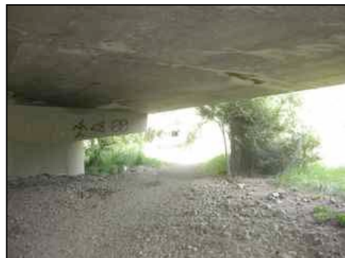
Figure 113. Trail under north structure
