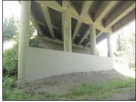
Figure 109. Support wall and side of north structure
