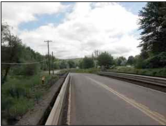
Figure 41. Highway 6 looking east
