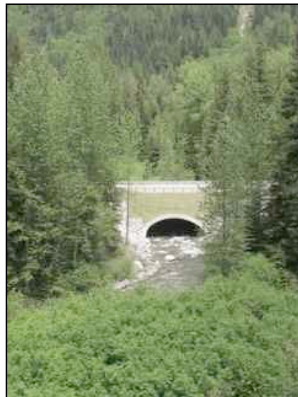
Figure 83. From eastbound lanes looking across median towards north structure
