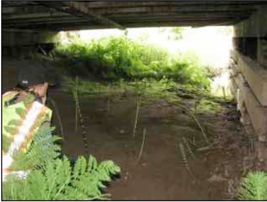
Figure 16. Stream bank under outside span
