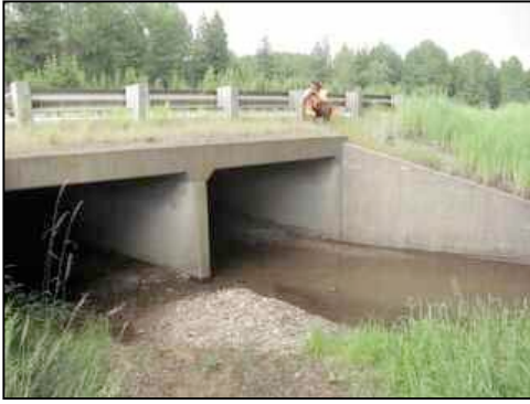
Figure 96. South side outlet
