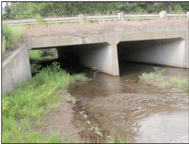
Figure 30. Example of a Class 2 Medium Culvert, I-90 WA © J. Kintsch & P. Cramer
