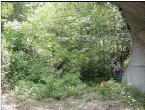
Figure 127. View from north structure outlet
