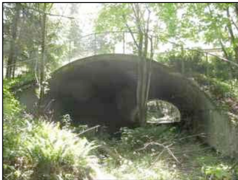
Figure 121. South structure entrance
