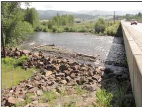
Figure 71. Riprap on east side of river outlet
