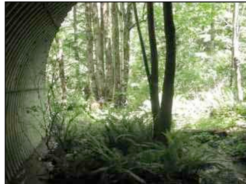
Figure 122. View from structure outlet
