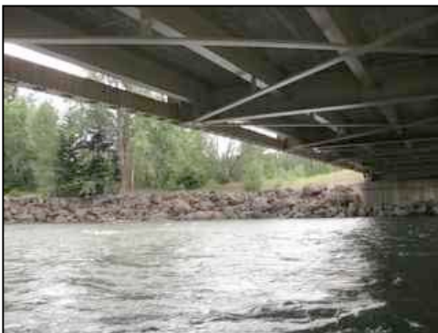
Figure 86. Riprap banks on east side of river
