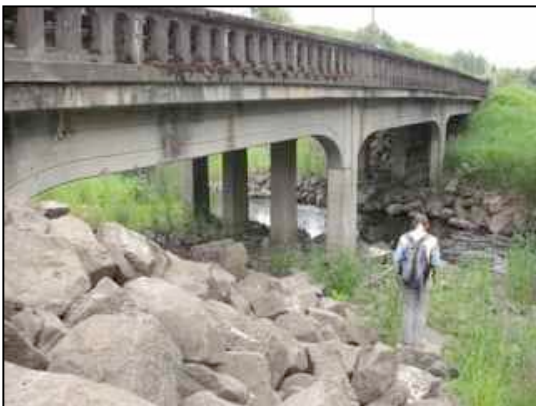
Figure 43. Bridge and riprap side slopes
