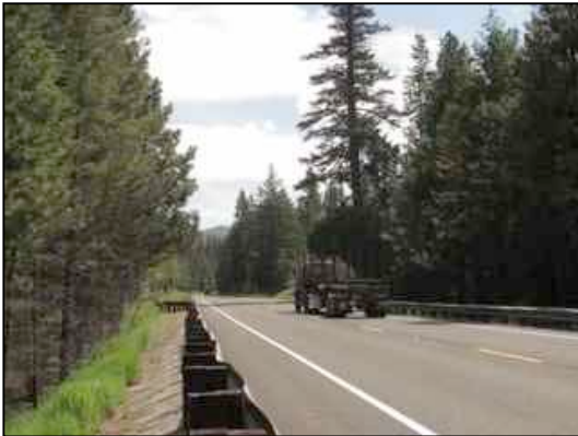
Figure 75. Roadway and adjacent forest
