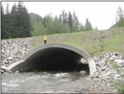
Figure 77. North-side structure outlet
