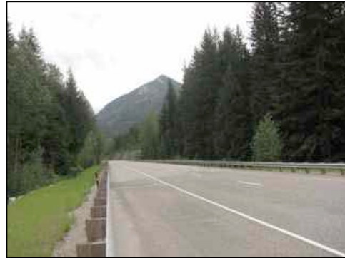
Figure 78. West bound lanes, looking east
