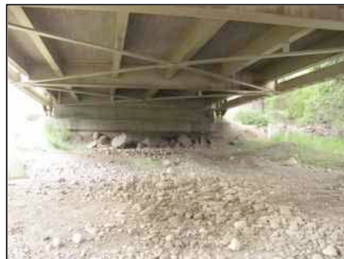
Figure 87. Dirt, rocky area on west side of river
