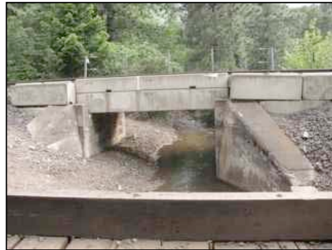
Figure 99. Adjacent culverts and infrastructure just beyond the south side of the interstate (under road & railroad)
