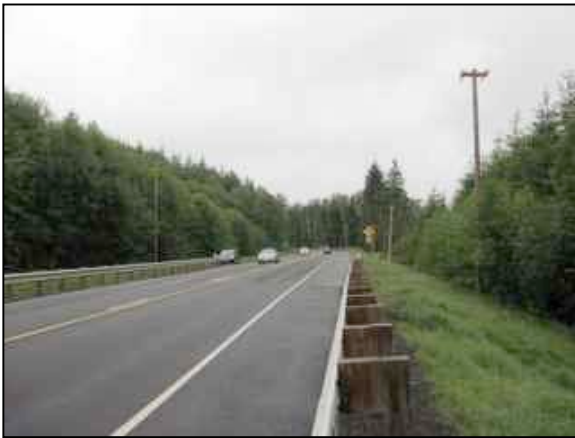
Figure 1. Rte 101 looking south
