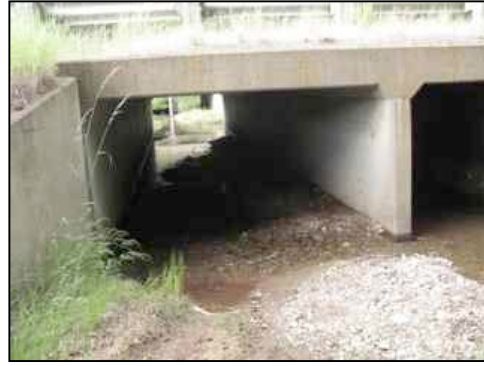
Figure 97. Semi-dry path through west chamber of south structure, with raccoon tracks
