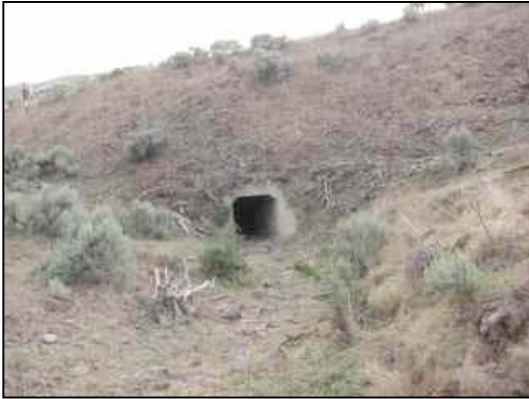
Figure 62. Box culvert at base of fill slope
