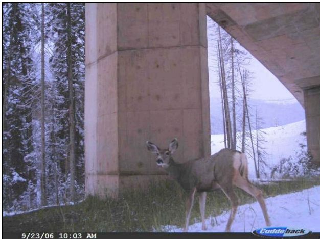
Figure 3. Multi-span bridge functioning as a crossing under I-70, Colorado © Center for Native Ecosystems, ECO-resolutions, LLC & CDOT
