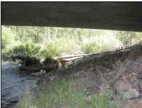
Figure 69. Side slope on west side of river
