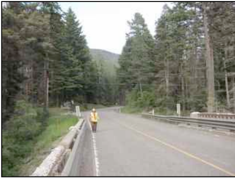
Figure 57. Roadway looking east
