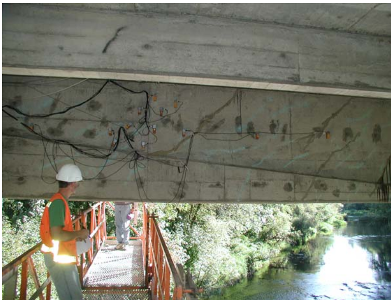
Acoustic emission testing at Banzer Bridge
