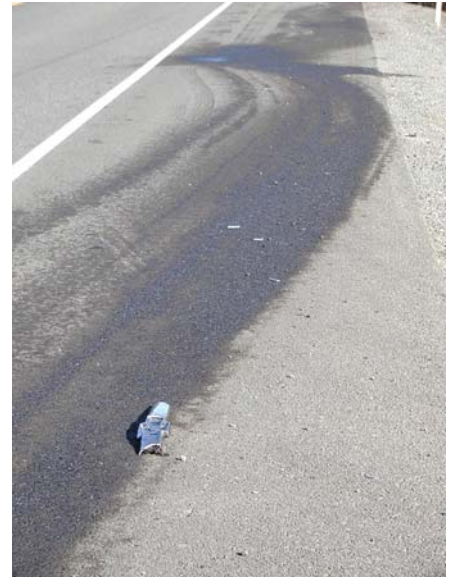
Trim pieces and transmission fluid from a truck that struck a deer on U.S. Highway 97 south of La Pine, Oregon
