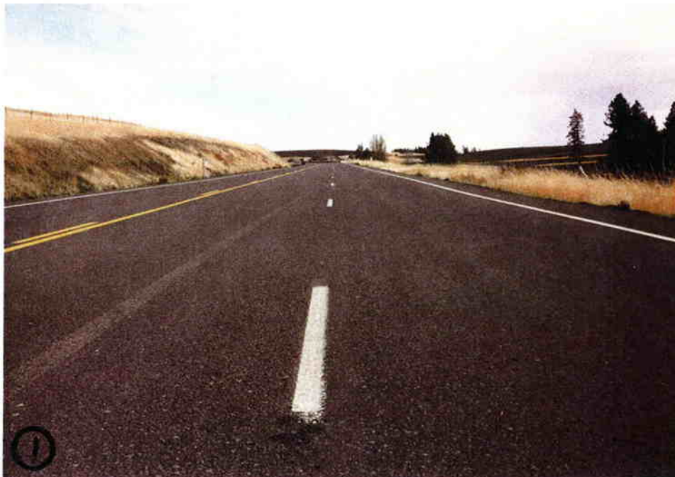
(b) Milepost 4.25 (looking South)
