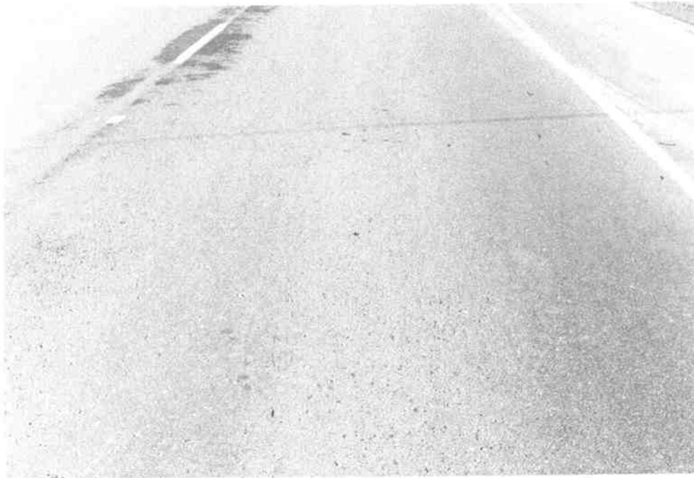
(a) Milepost 285.88, Southbound
