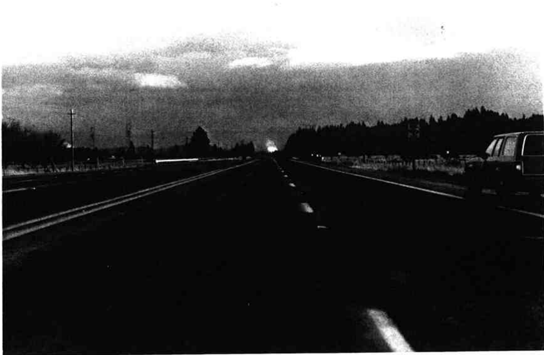
(b) Station 1206+24.0, Eastbound travel lane
