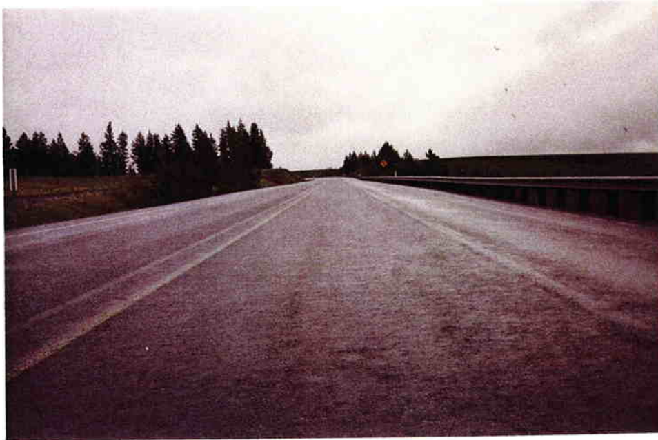
(a) Milepost 5.30 (looking East)
