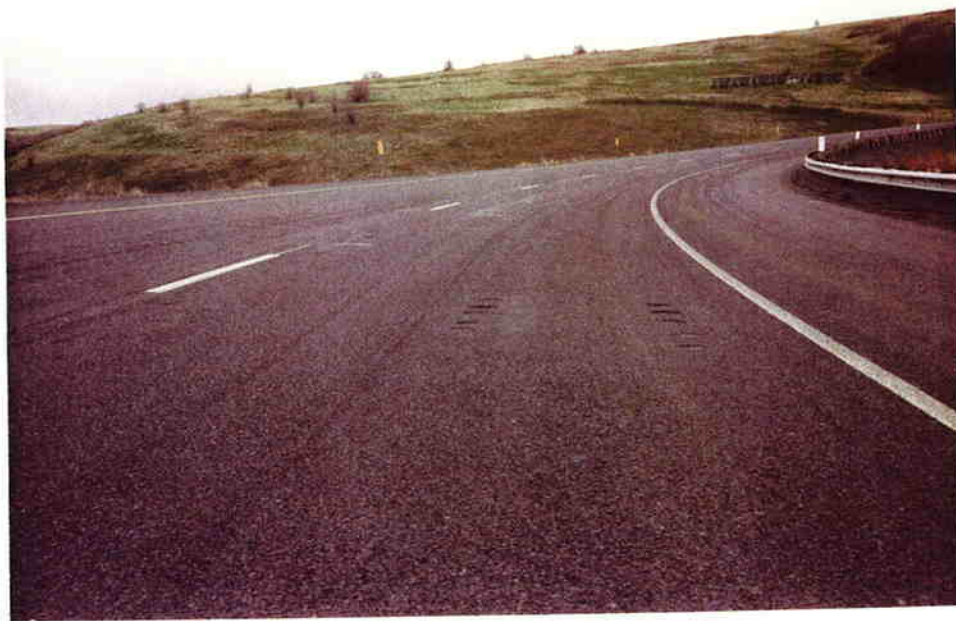
(c) Eastbound, MP 223.64 (looking East)
