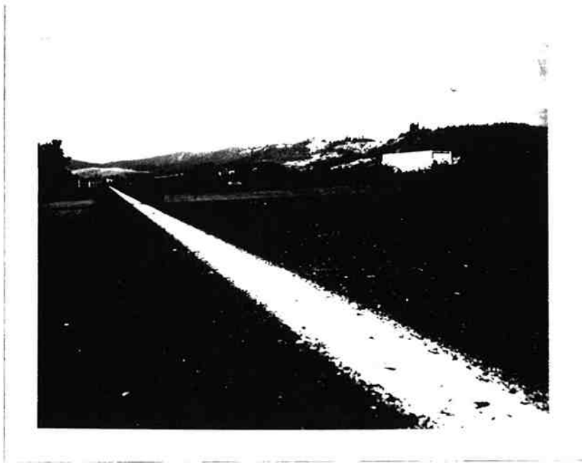
(a) Milepost 151.70, Northbound Lanes
