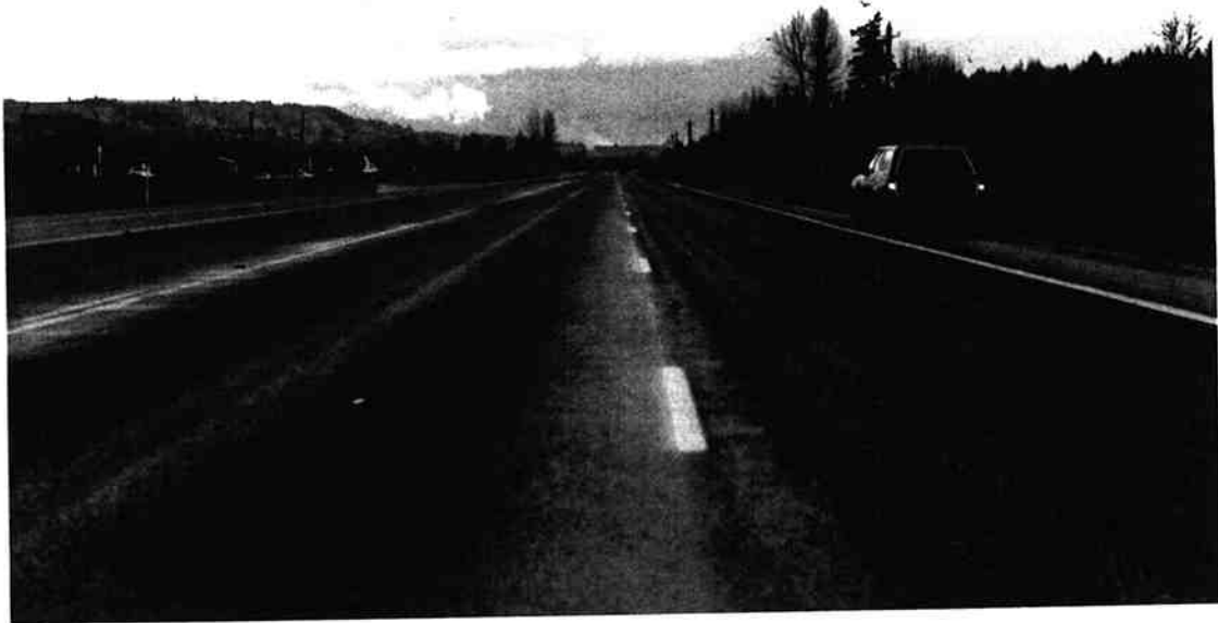
(a) Station 1130+00, Eastbound
