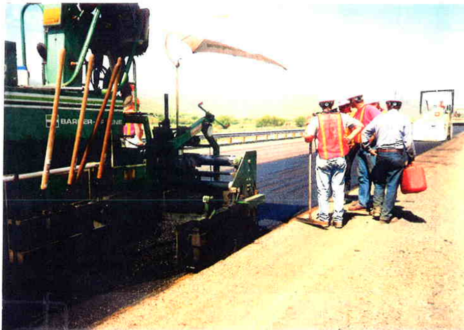
Figure 2.13 Rolling and compacting of recycled mix behind paver.
