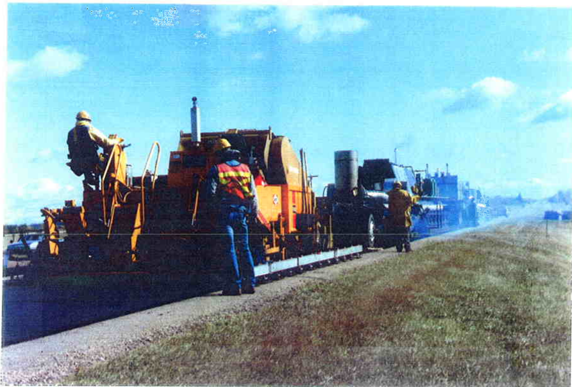
Figure 2.26 Recycled mat just behind screed. (Photo courtesy of ARTEC.)
