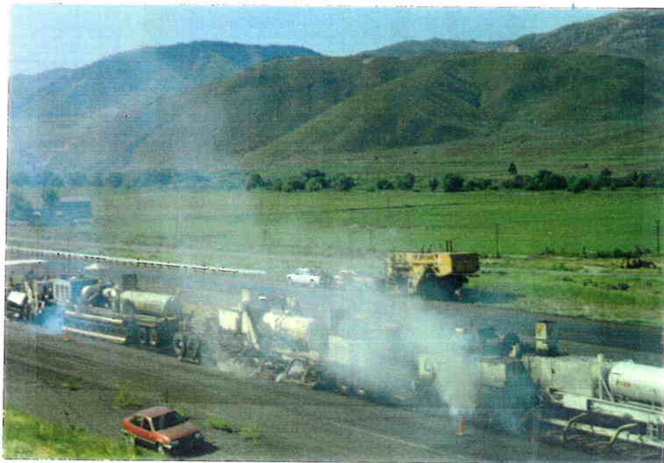
Figure 3.43 Close-up of Pyrotech-Arttec recycling train used on Durkee-Lime HIR project.
