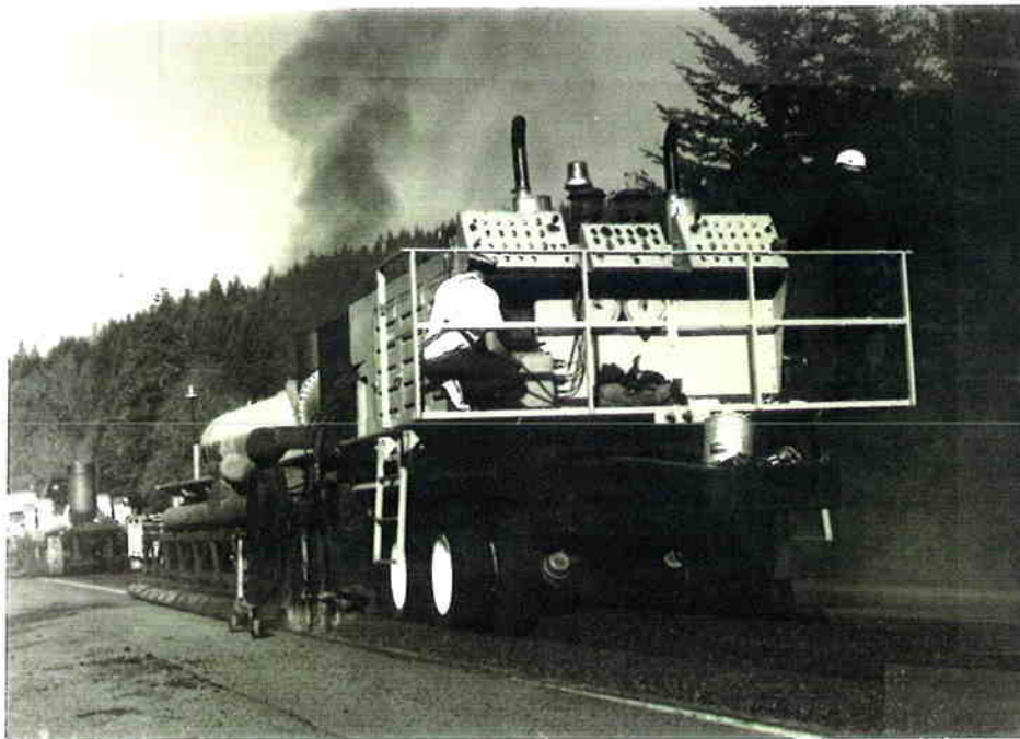
Figure 2.24 View of recycled mixture windrow after passing through pugmill.
