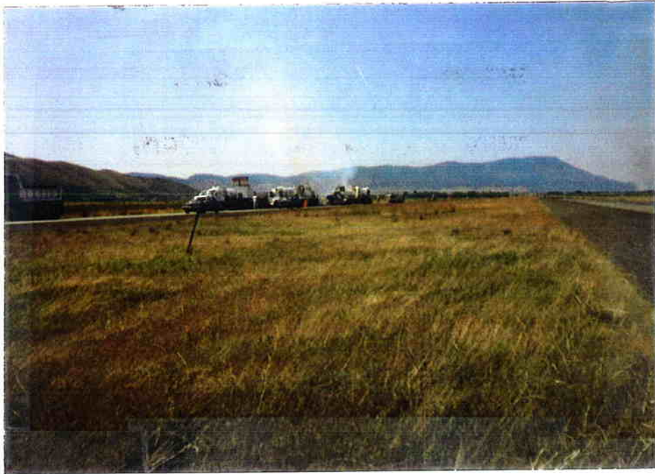
Figure 2.2 Pyrotech PYROPAVER 300E recycling train in operation.
