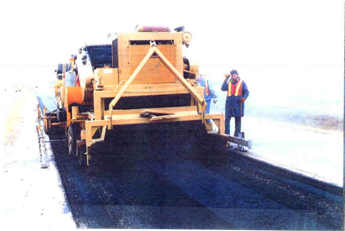
Figure 2.25 Windrow of recycled mixture entering pickup paver. (Photo courtesy of ARTEC.)
