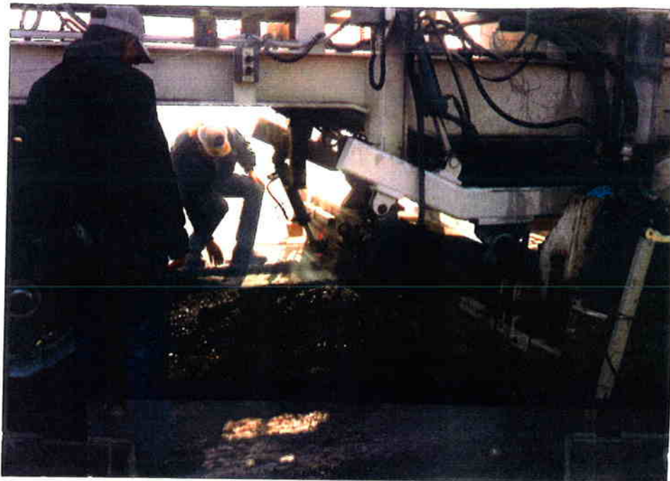
Figure 2.11 Close-up of second miller/grinder, just before RAP and virgin mix are combined.
