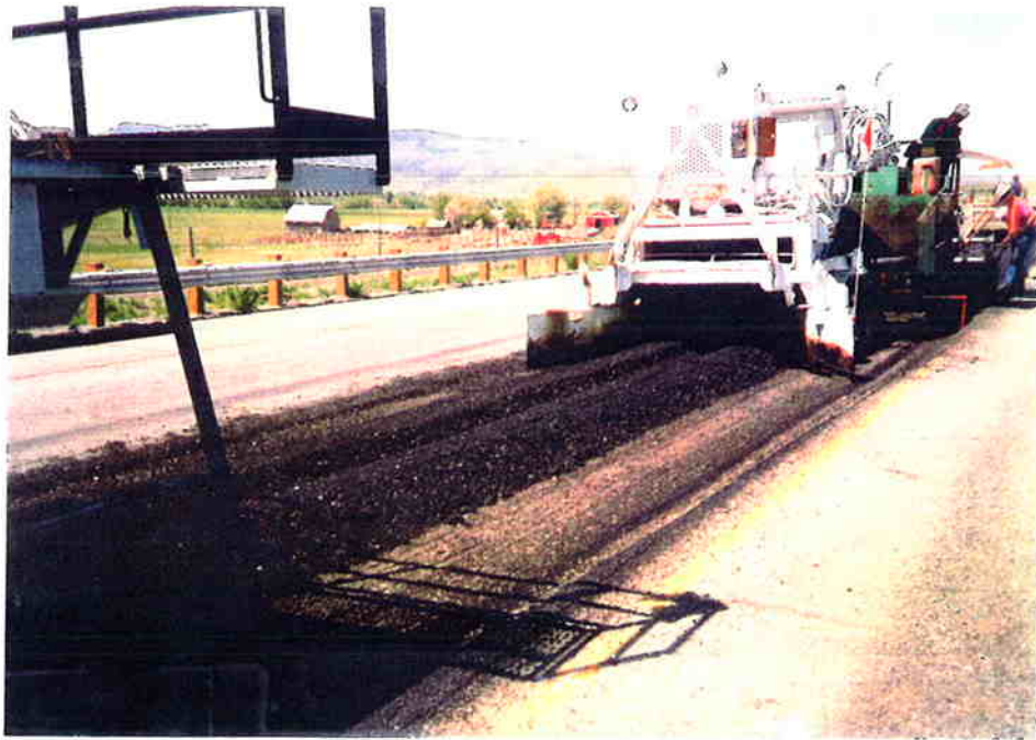
Figure 2.12 Combined RAP/virgin mix as it enters the pugmill.
