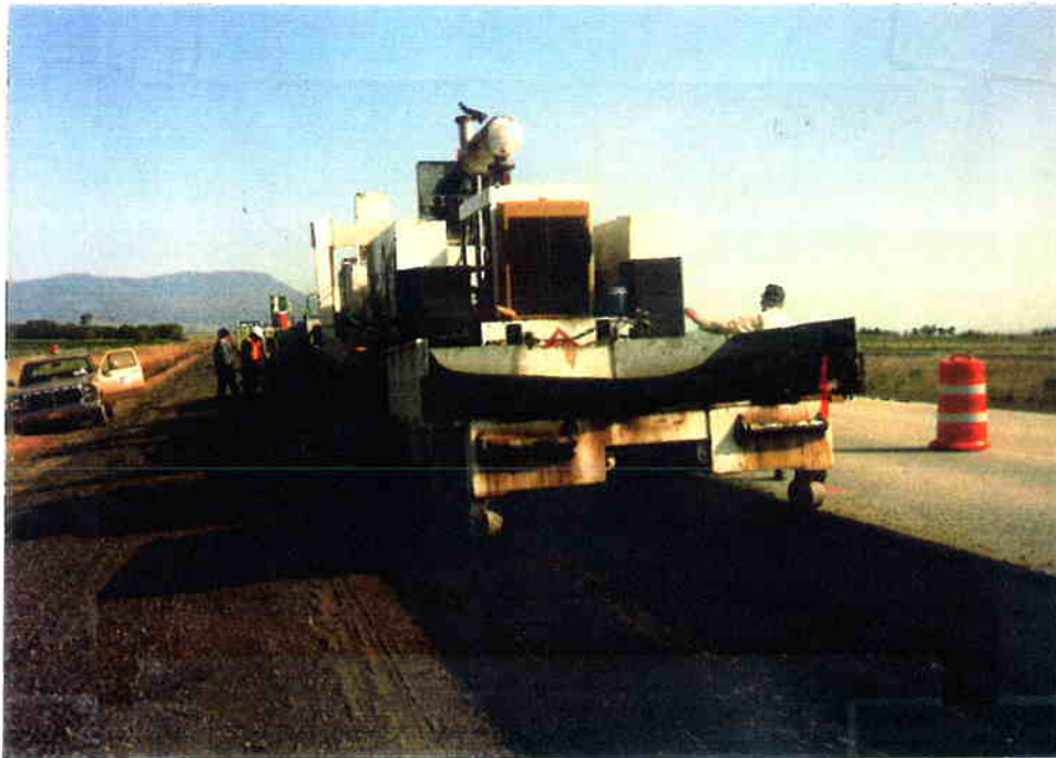
Figure 2.9 Hopper at the front of unit 2 for addition of virgin mix.
