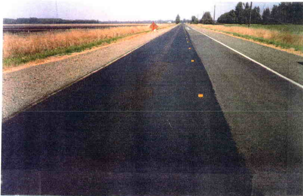
Figure 3.27 Raveled section after HIR.
