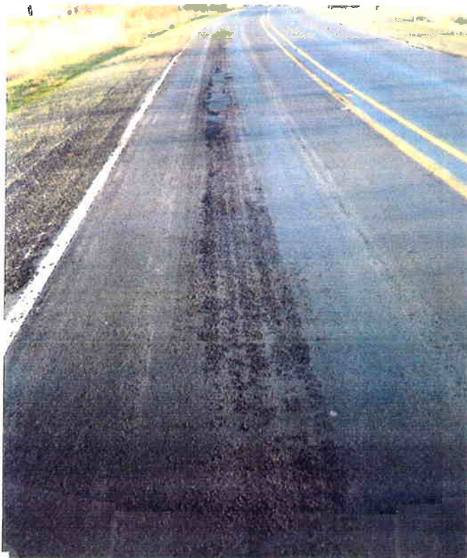
Figure 3.29 Freshly sand sealed area with visible patched area.
