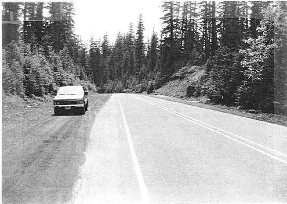
Figure 3.15 Good section near mile point 7.4.
