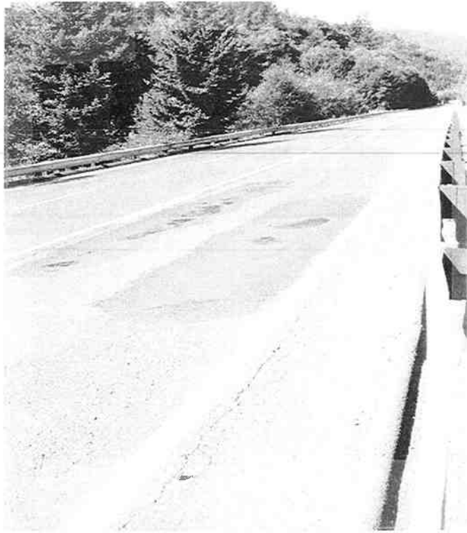
Figure 3.40 Section with blade patching in the non-HIR lane and good looking HIR lanes.
