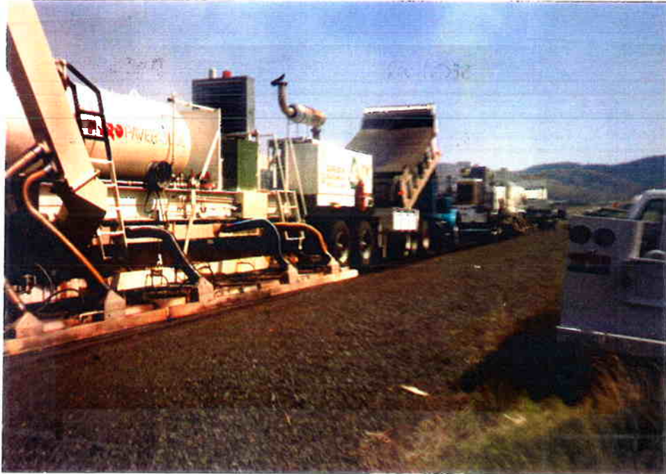
Figure 2.10 Truck dumping virgin mix into hopper.
