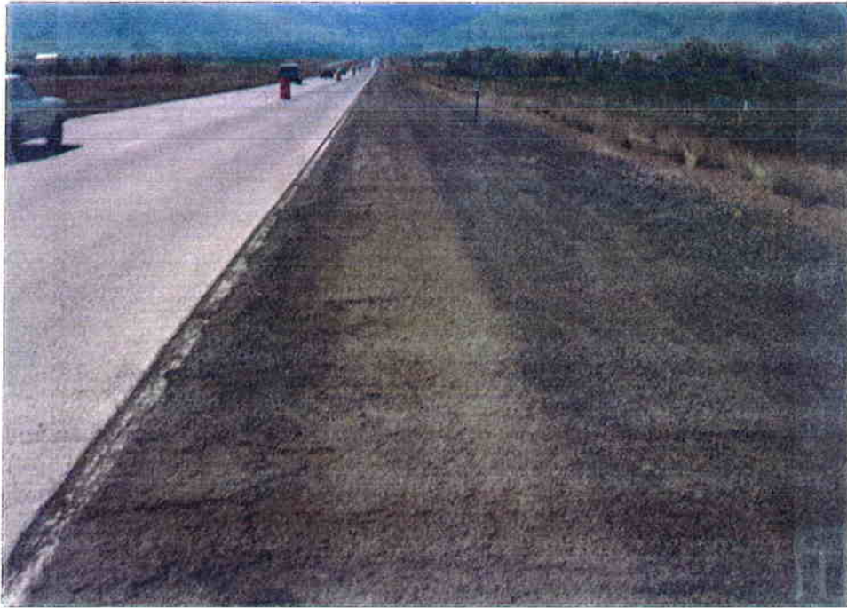
Figure 3.2 Example of I-84 shoulder pavement prior to HIR.
