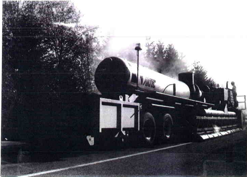
Figure 2.19 Hopper at front of unit 2 for addition of virgin mix.
