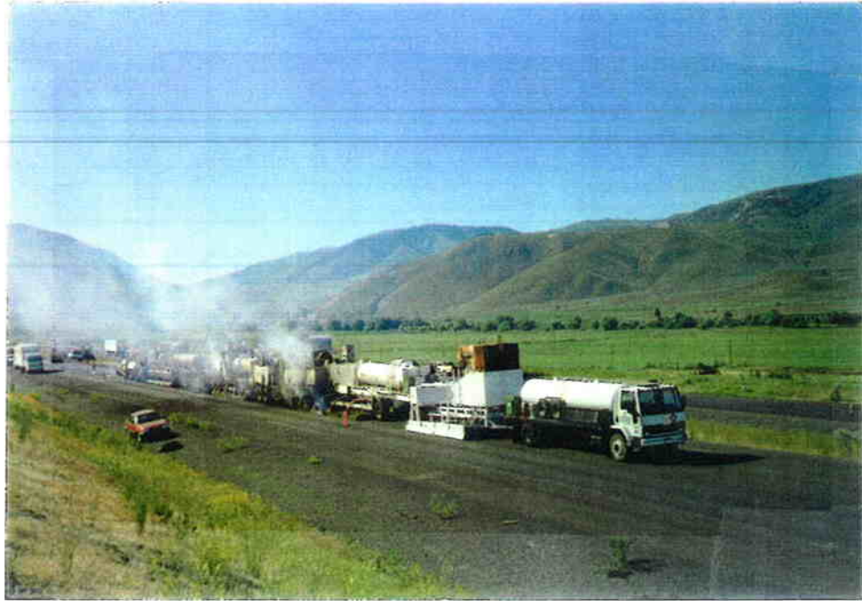
Figure 3.42 Unique Pyrotech-Arttec recycling train used on Durkee-Lime HIR project.
