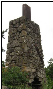
Figure 3.33: Crag Rats Club House Chimney
