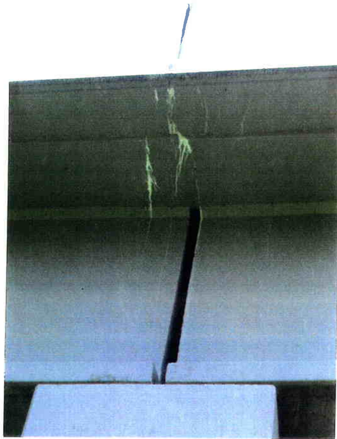
Figure 3.1: Sealed Cracks at the North Side of Bent 3
