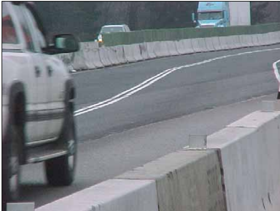
Figure 1.1: Typical concrete barrier used for a lane shift in an Oregon work zone
