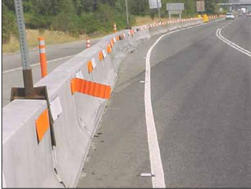
Figure 5.2: Panel detachment from the barrier at the Coast Fork Willamette River Bridge project
