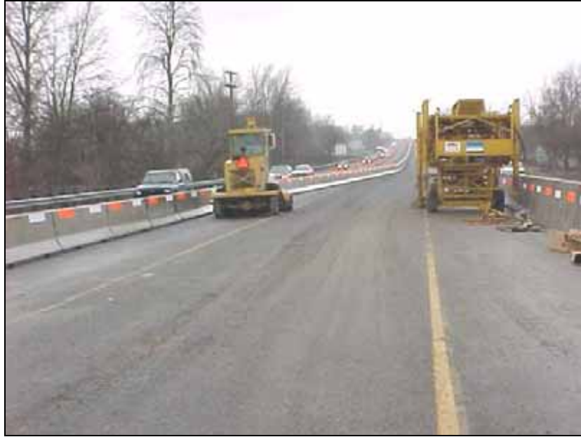
Figure 3.4: Approaching lane shift at Medford Viaduct
