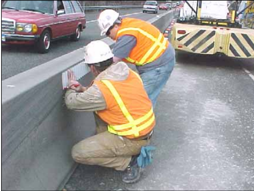
Figure 4.2: Marking holes for drilling
