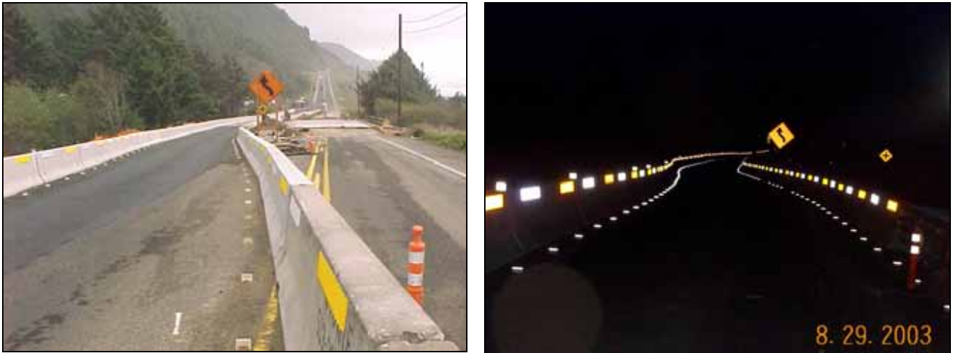
Figure 6.1: Day and night comparison of Bob Creek Bridge site looking southbound
