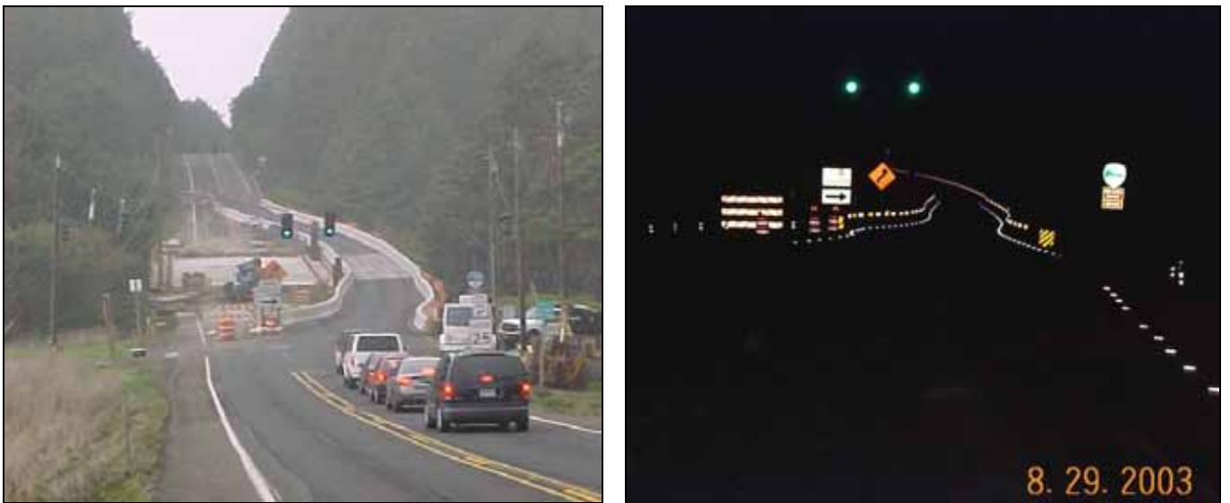
Figure 6.2: Day and night comparison of Bob Creek Bridge site looking northbound
