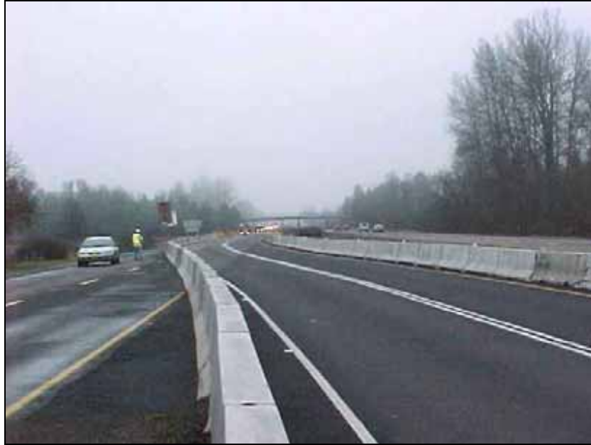
Figure 3.2: Approaching lane shift at the Coast Fork Willamette River Bridge
