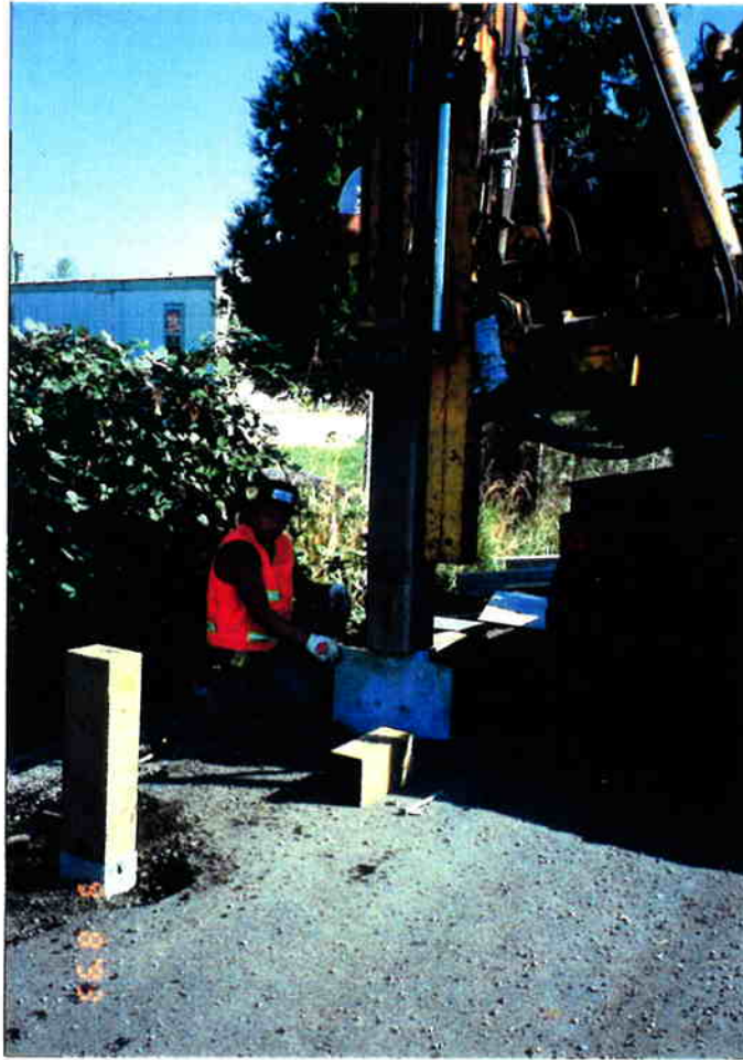
Figure A.1: ET-2000 Soil Plate and Steel Foundation Tube Installation.
