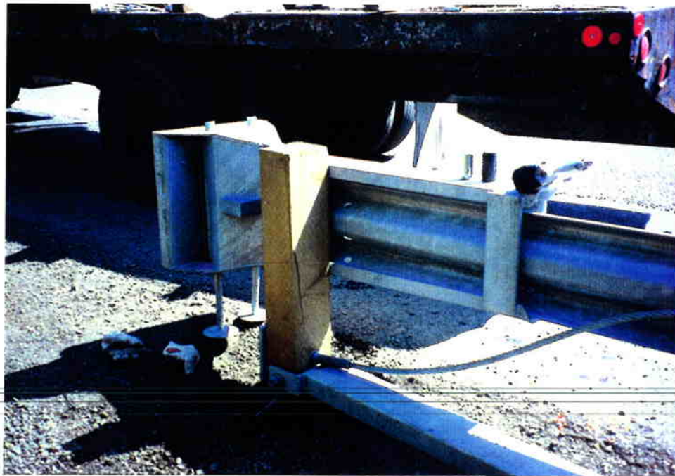
Figure A.3: ET-2000 Guardrail Extruder Head, Offset Strut, and Cable Assembly Installation.
