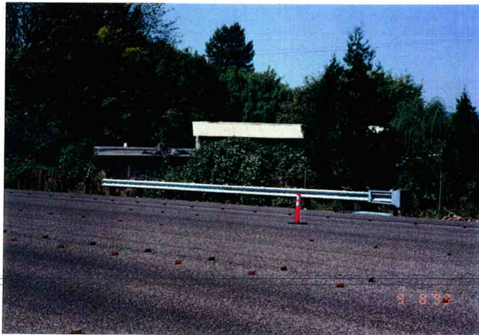
Figure A.5: ET-2000 Extruder Guardrail End-Terminal; unit installation completed.
