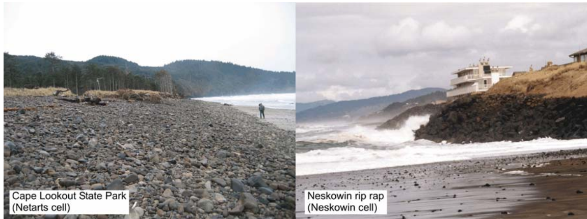
Figure 3.4: Comparison of a dynamic revetment constructed at Cape Lookout State Park (left) versus a conventional riprap revetment constructed at Neskowin (right)
