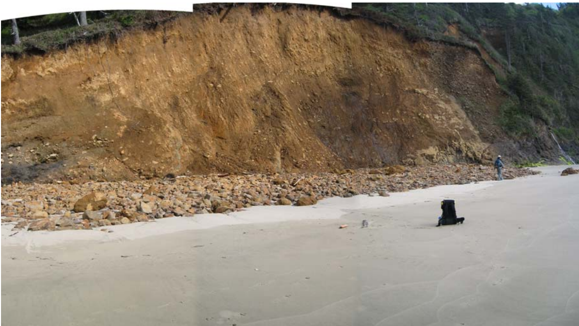
Figure 5.1: A landslide that occurred early in 2003 on the north side of Cape Lookout and adjacent to Cape Lookout State Park. Such events periodically introduce significant quantities of coarse material to the coastal zone where it is then redistributed along the shore to form cobble berms.
