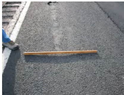
Figure 2.18: Rutting on I-90 in Washington State attributed to stripping of the underlying layer
