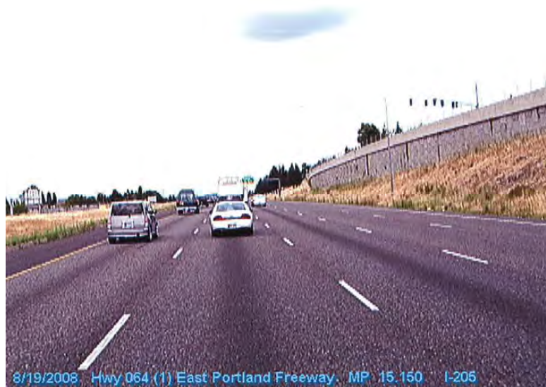
Figure 3.1: I-205 MP 15.15 showing pavement in good condition.
