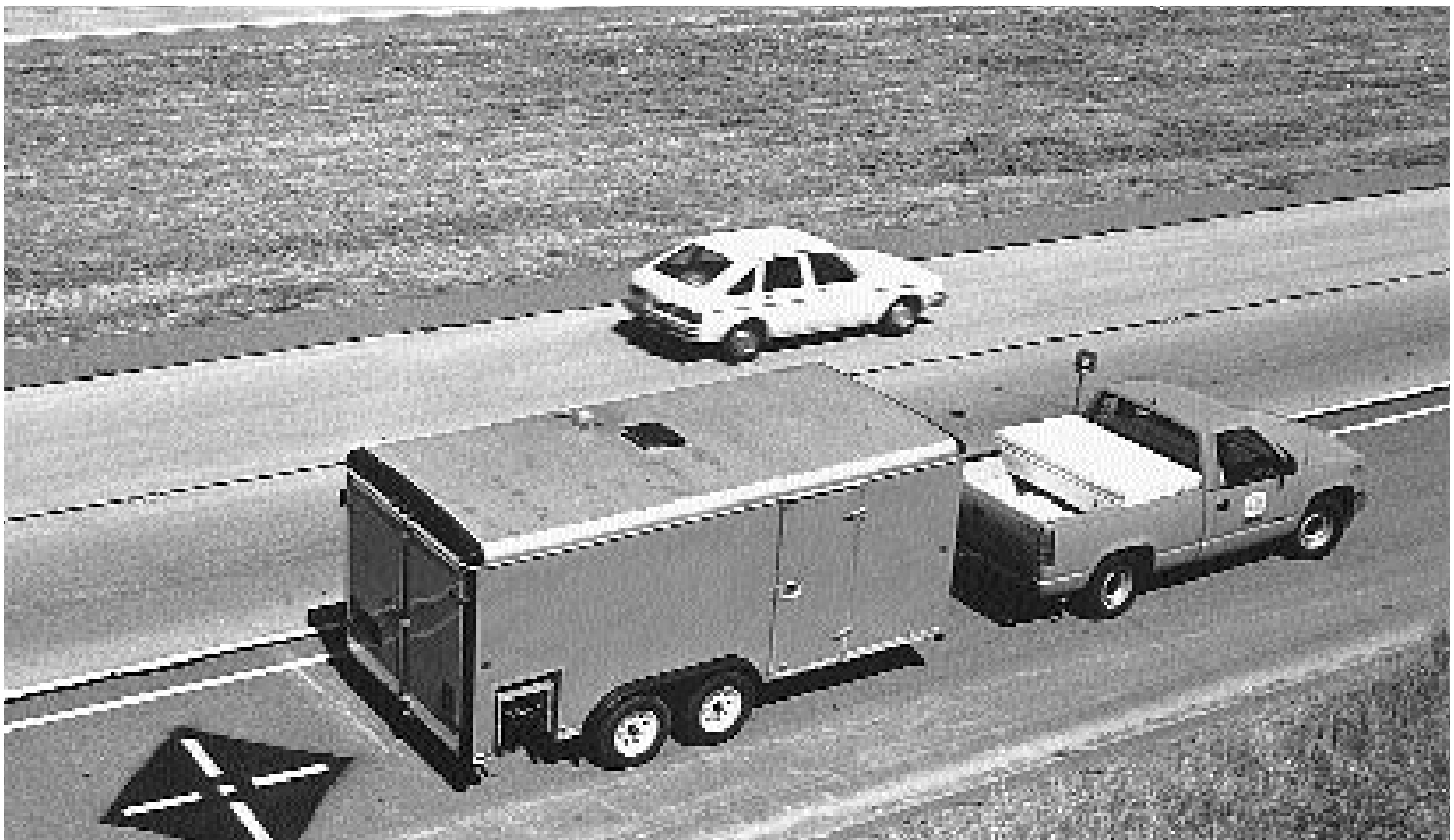
Robotic System for Sign Stenciling in operation.
