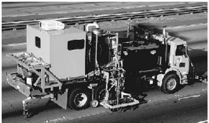
Crack sealing machine prototype testing, District 3 (Marysville)
