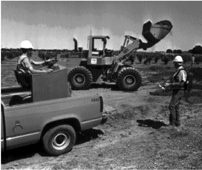
TAMER equipment in operation. Both of the methods shown, the backpack unit and stationary console, are available for remote operation.
