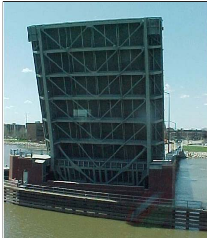
Figure 4. Underside of west leaf of Main Street bridge in open position.
