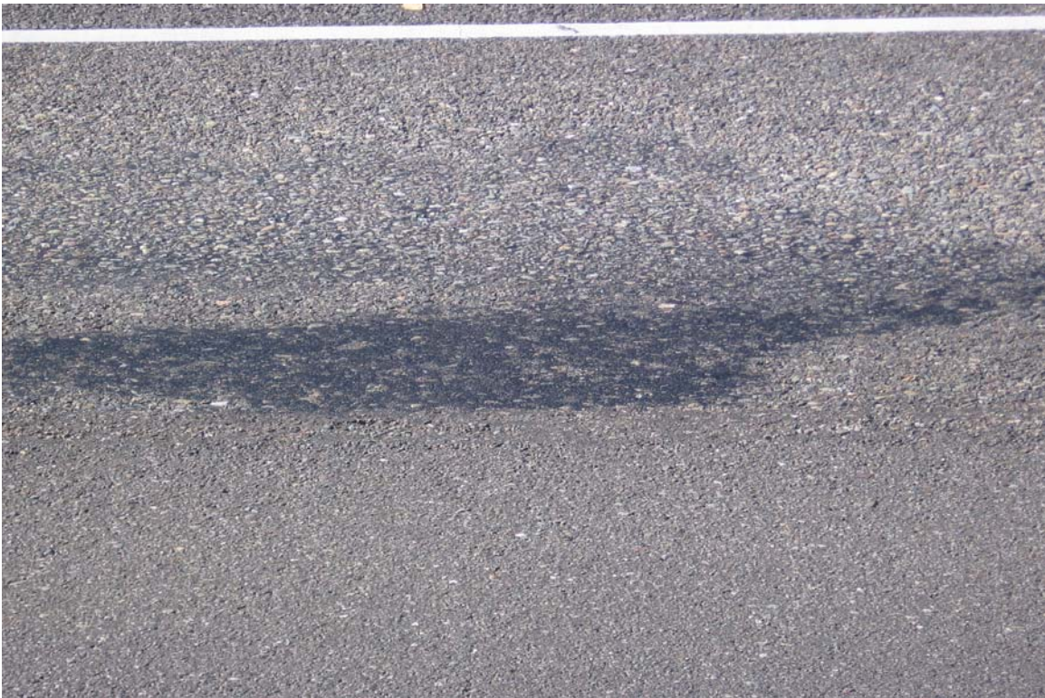
Figure D-1.18: Bleeding Of Binder, a Common Sight in This Part of the State
