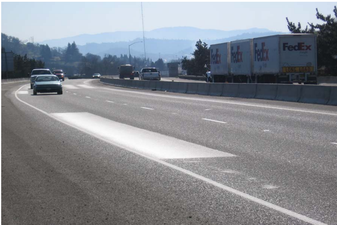
Figure D-1.15: Representative Example of the Numerous Patches Found In This Project
