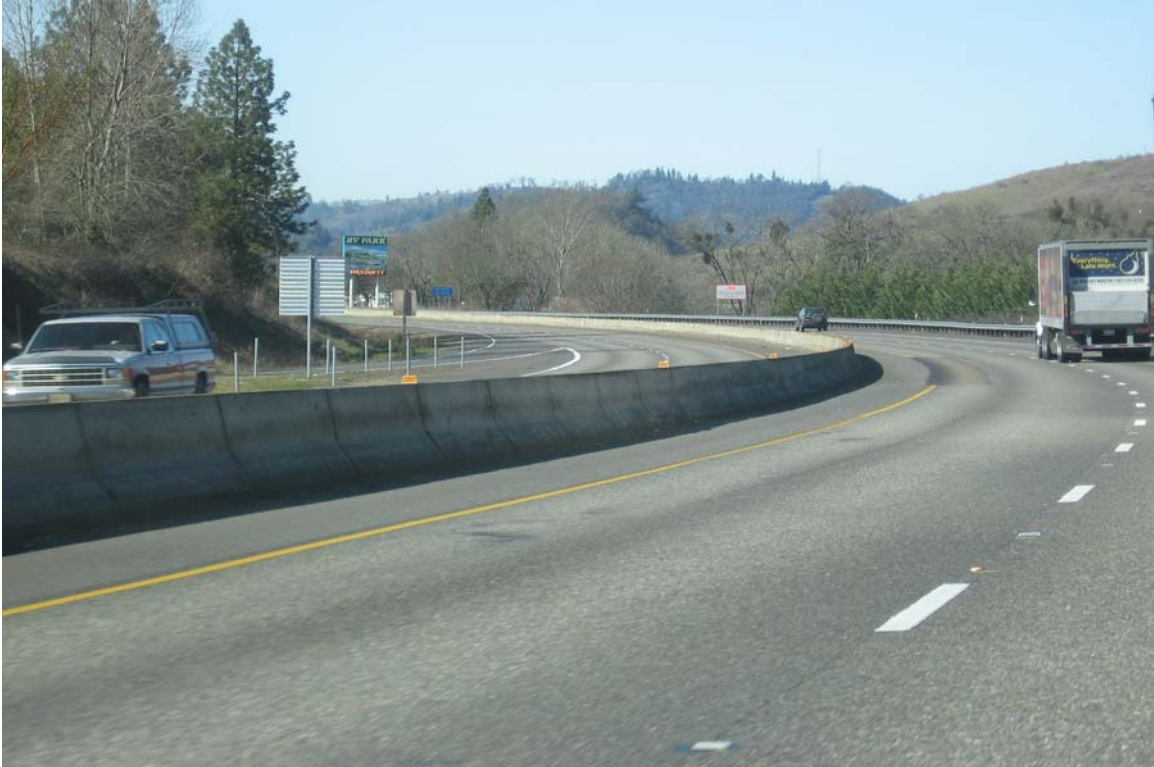
Figure D-1.27: Example of a Patch Found On the Inside Lane of the Pavement Section
