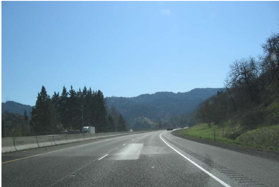
Figure D-1.19: Patch Visible In the Wheel Path of the Outside Lane
