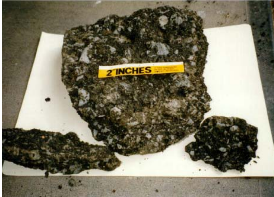
Figure A-3.3: Example of Badly Stripped AC 28 and AC 14 Courses.
