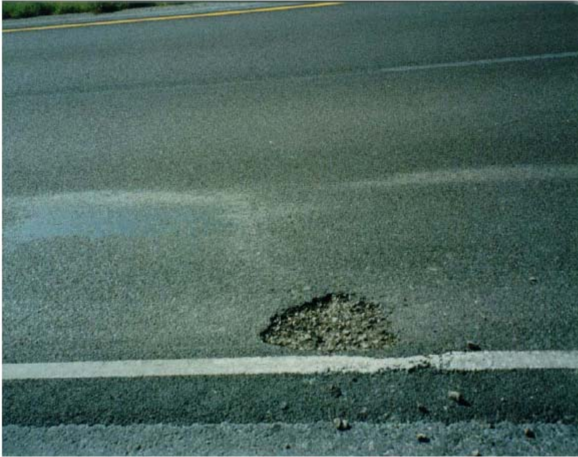
Figure A-3.1: Three Stages of Stripping: White Stains, Flushing, and Pothole (After Kandhal 2001 )
