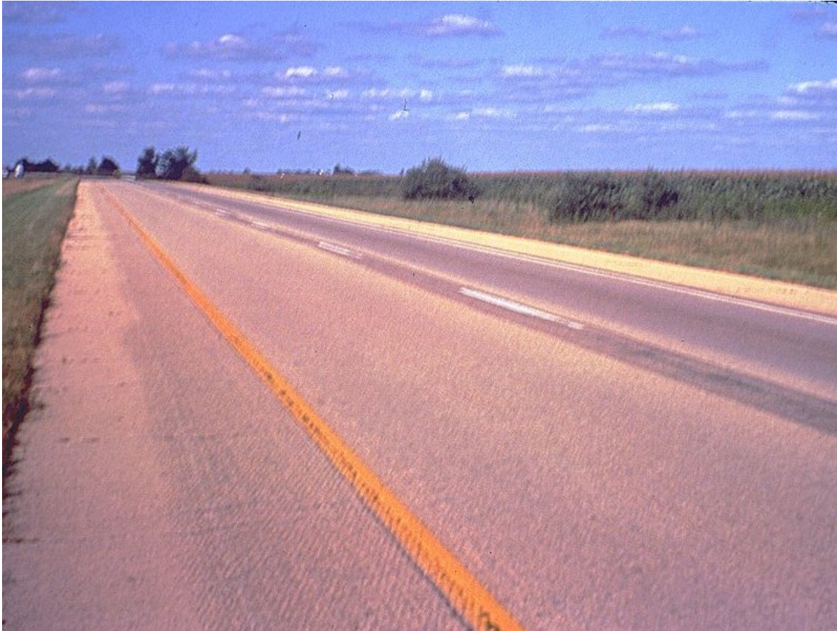
Figure A-5.2: Properly Milled Pavement Surface
