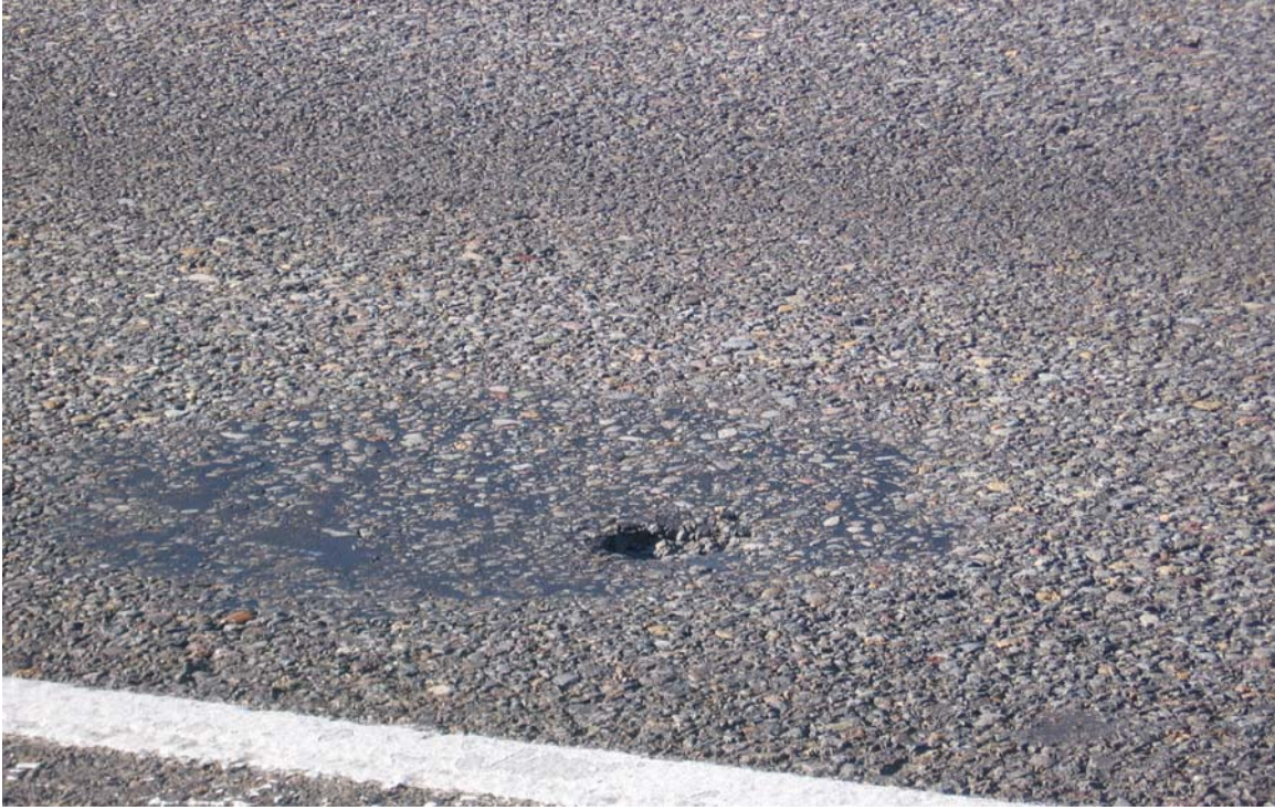
Figure D-1.10: A Pot Hole with Some Bleeding
