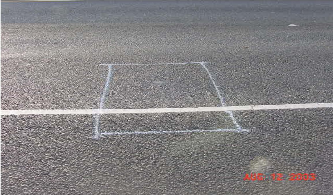
Figure C-1.1: First Trench Cut in an Area of Observed Distress
