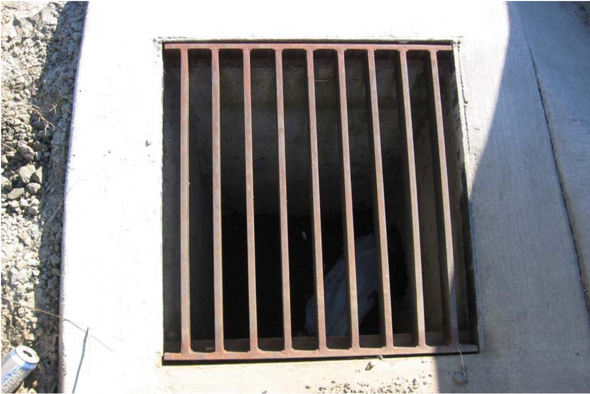
Figure D-1.30: Properly Maintained Drain with No Clogging
