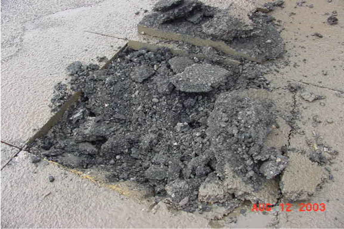
Figure C-1.2: Unstable Mix from the Trench
