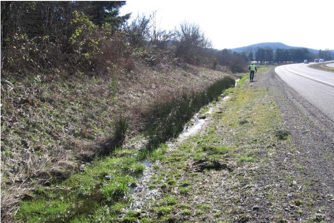
Figure D-1.11: Very Low Flow Rate of Water in This Ditch Has Allowed the Growth of Algae and Other Plants Commonly Found In Ponds
