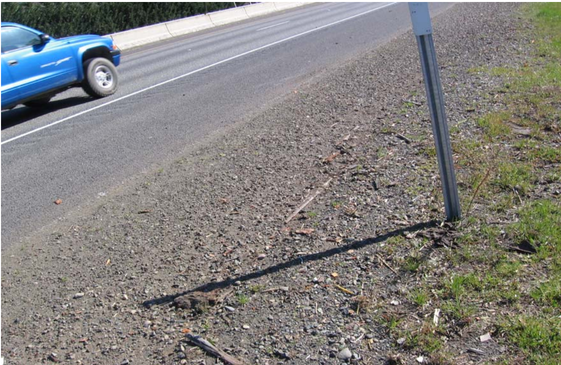
Figure D-1.24: Inadequate Slope and Vegetation Growth Seen Close To the Pavement at MP 111
