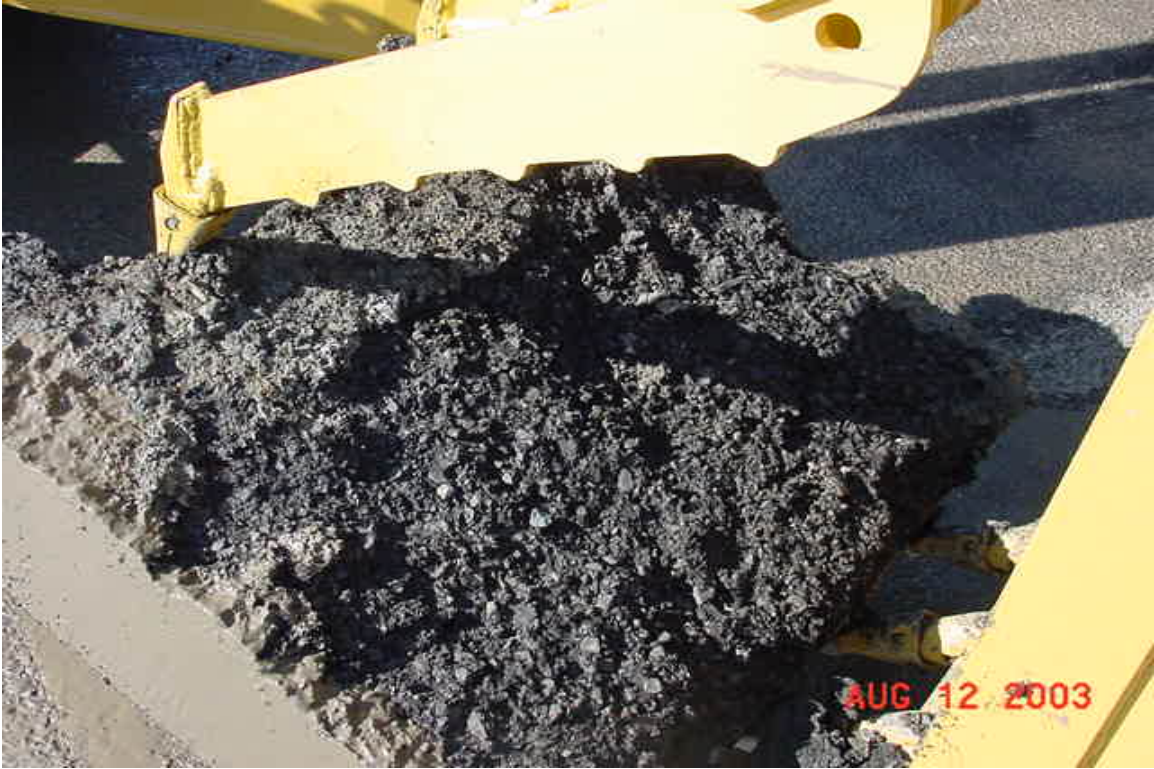
Figure C-1.5: HMA Layer Trenching With Back Hoe in Second Trench
