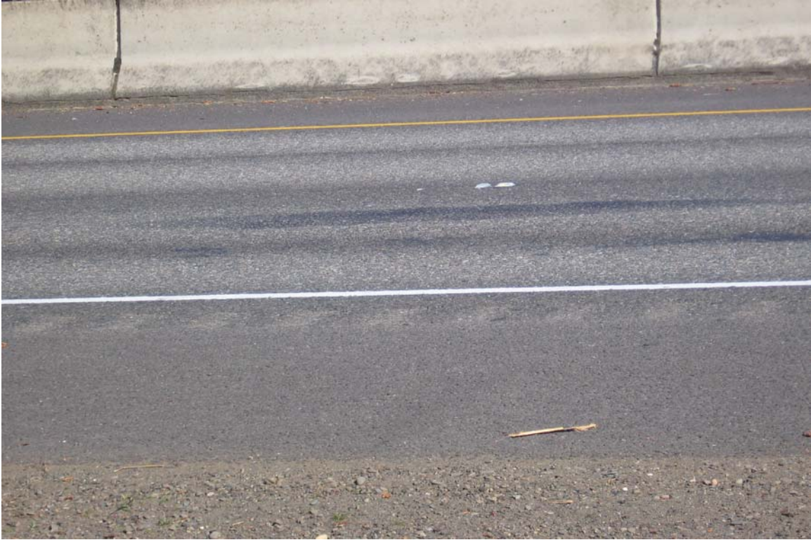
Figure D-1.23: Bleeding Observed On the Pavement Section Adjacent To the Rest Area at MP 111
