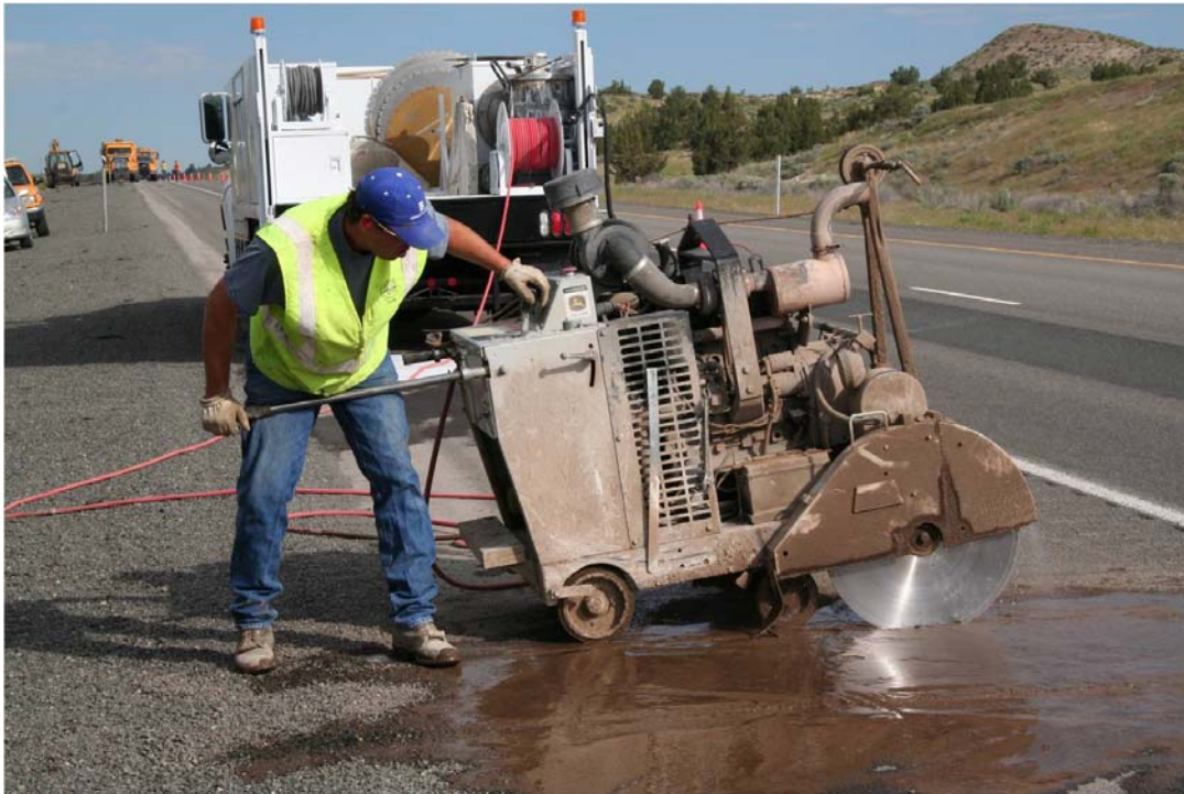
Figure 3.1: Cutting the Bound Layers for the Trenching Operation.
