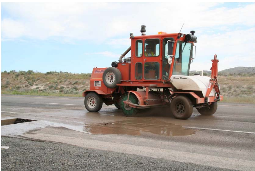
Figure 3.2: Sweeping the Surface over the Saw Cuts.
