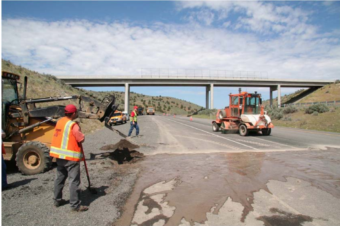
Figure 3.3: Using a Backhoe with Fork Attachment to Remove Bound Material.
