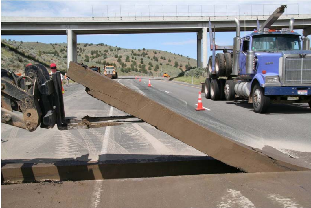
Figure 3.5: Excavation of the Travel Lane Slab with SMA Wearing Course Intact.
