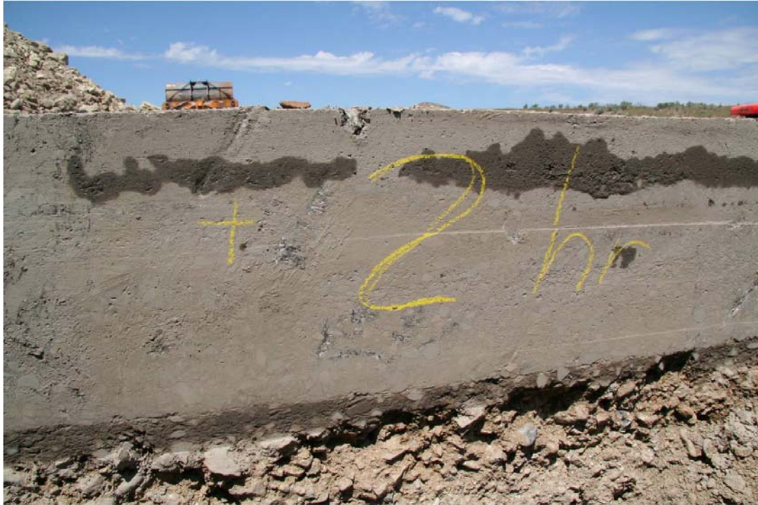
Figure 3.18: Uphill Face of Trench at MP 324.9 Approximately Two Hours After Excavation.
