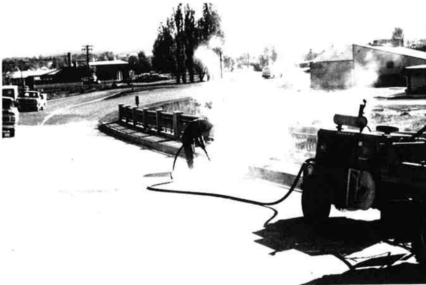
Figure 5. Final deck cleaning by sandblasting.
