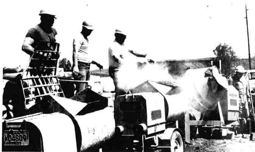
Figure 9. Adding aggregate into mixers.
