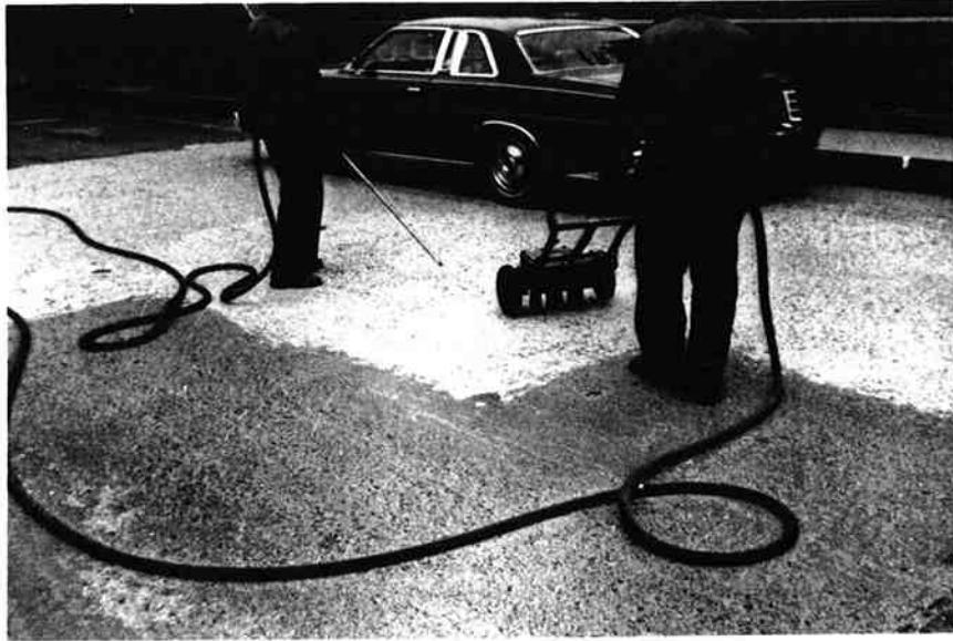
Figure 4. Deck preparation by scabbling.
