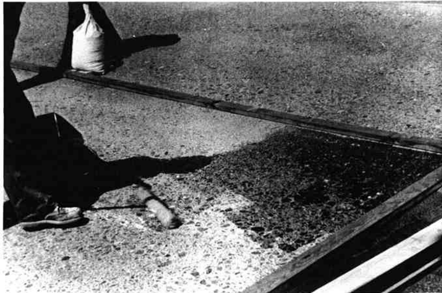
Figure 12. Tack coat application.
