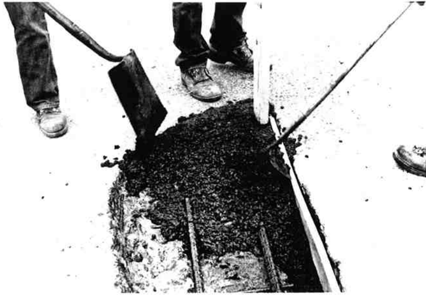
Figure 20. Placing and compacting polymer concrete patch.
