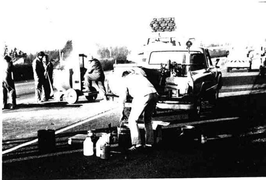
Figure 18. Resin formulation at job site.
