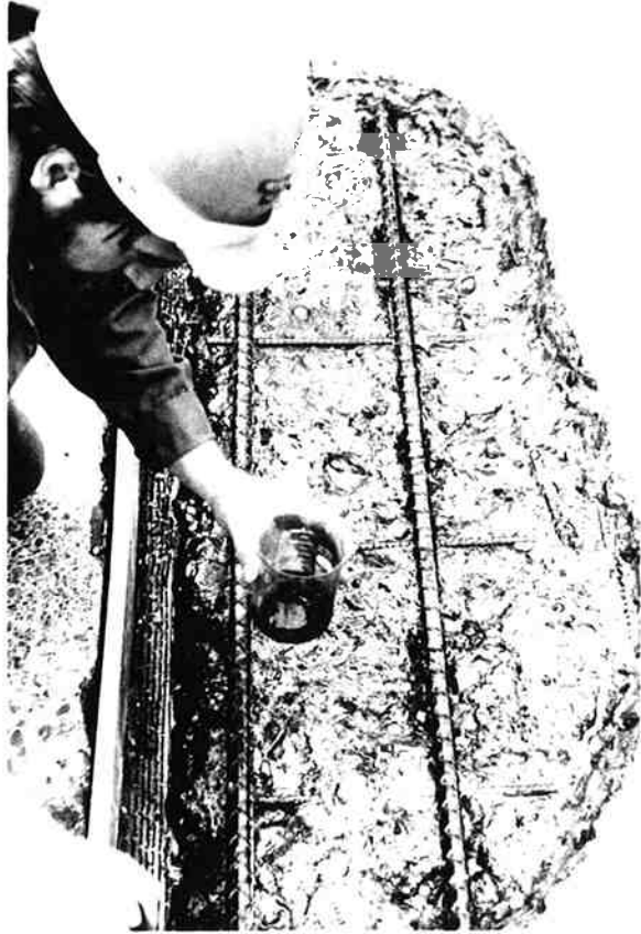
Figure 19. Tack coat application.
