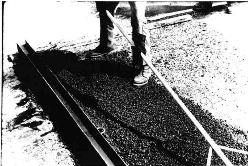
Figure 14. Spreading polymer concrete before screed.
