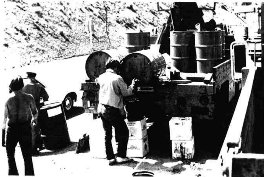
Figure 7. Withdrawing resin into pre-calibrated containers.
