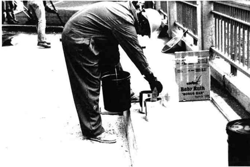
Figure 11. Adding initiator to tack coat resin.
