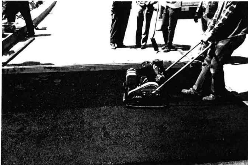
Figure 15. Consolidating polymer concrete.
