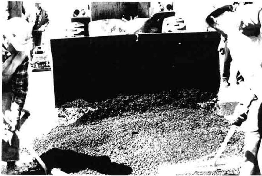
Figure 13. Polymer concrete deposited on deck.
