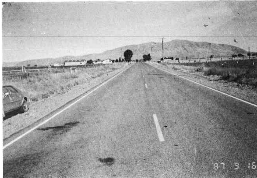
Figure B.5 - Typical pavement surface condition of the US 97 - OR 39 (Lower Klamath Hwy) project. Photo was taken at MP 3.65 looking ahead on line on September 16, 1987. Surface is chip sealed.
