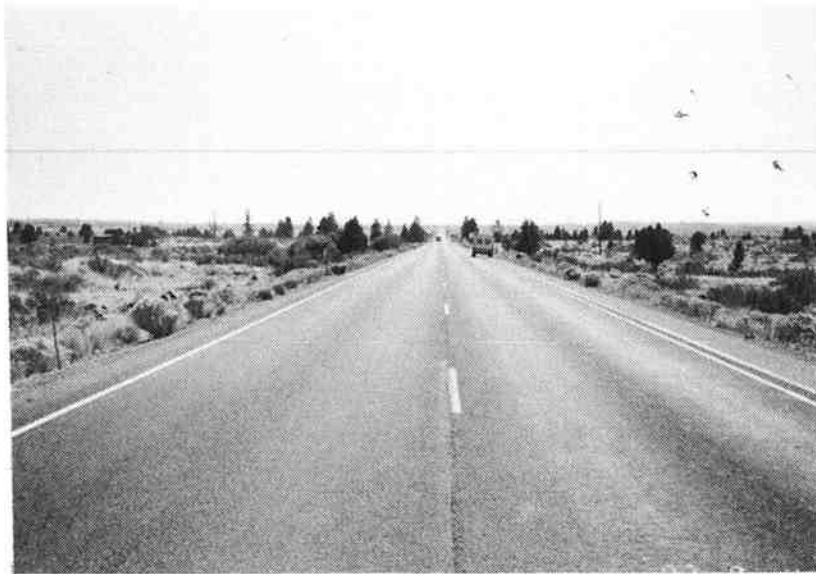
Figure B.1 - Typical pavement surface condition of the MP 79.2 - Wasco Co. (Warm Springs) project. Photo was taken at MP 89.7 looking ahead on line on September 4, 1987. Surface is chip sealed.
