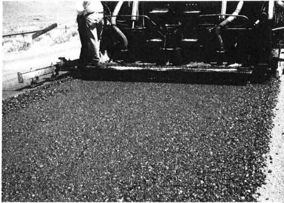
a) Laydown with Paving Machine
