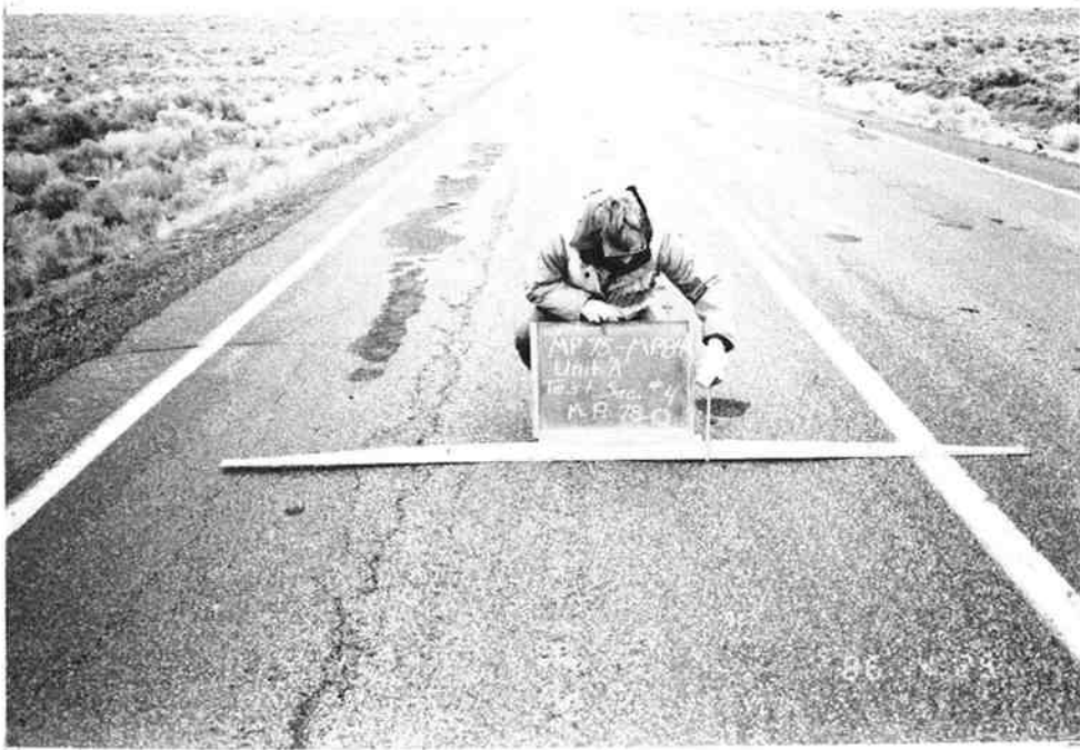
a) Central Oregon Highway, Unit A (Rated "Very Poor")
