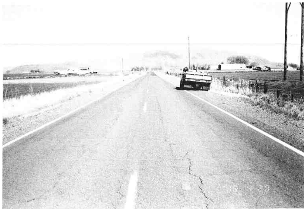
b) Ochoco Highway, Unit E (Rated "Very Poor")
