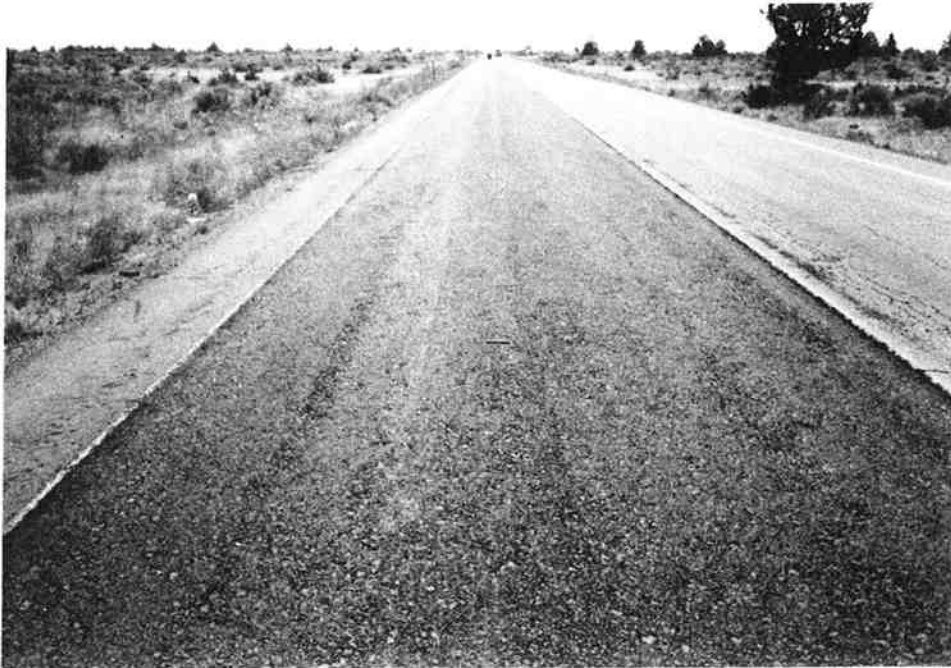
a) After Initial Compaction
