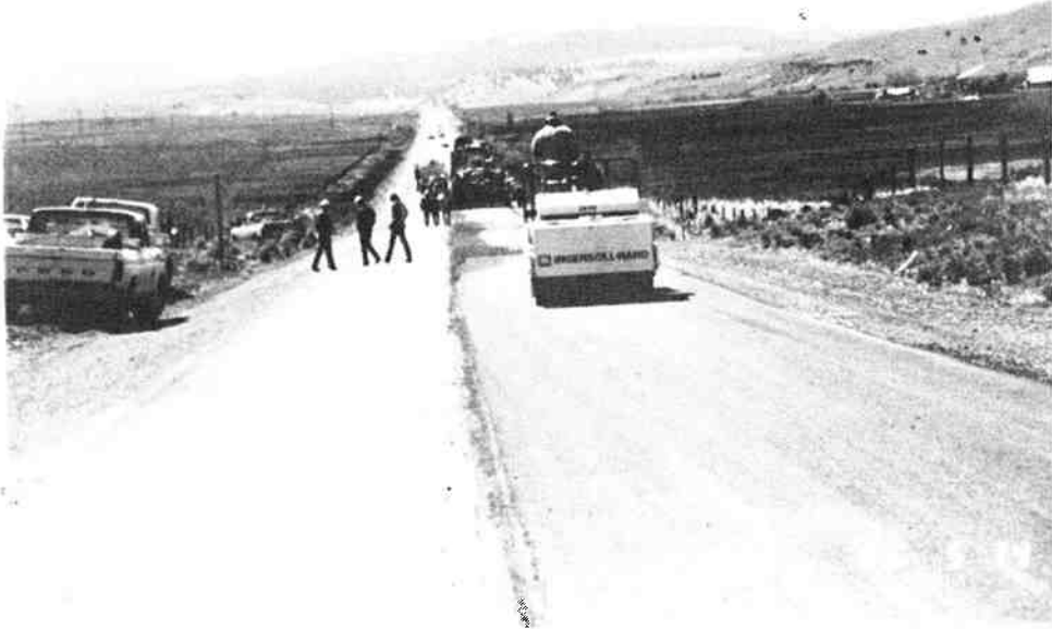
a) Initial Compaction
