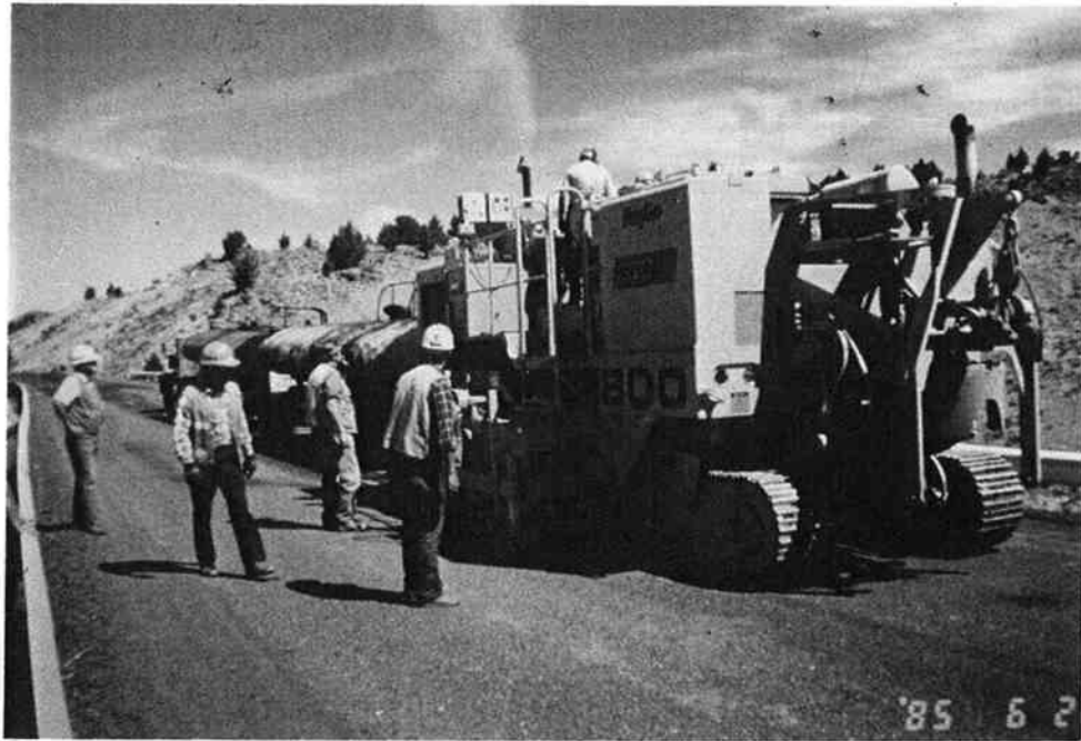
a) Milling and Mixing Operation
