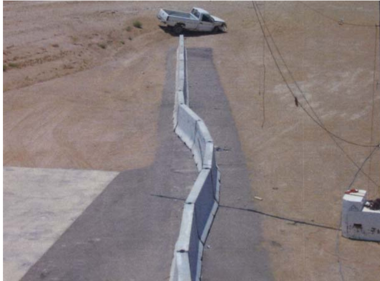
Figure 3.4: Tall F-shape barrier following Crash Test 2
