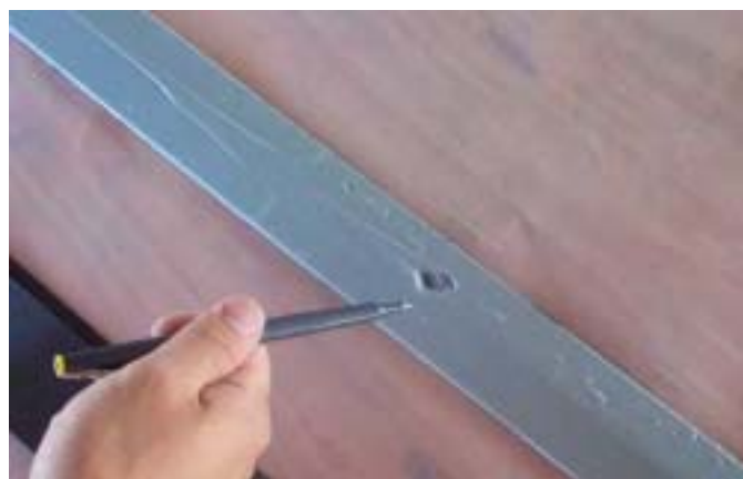
Figure 3-31: Formation of Void During Putty Application
