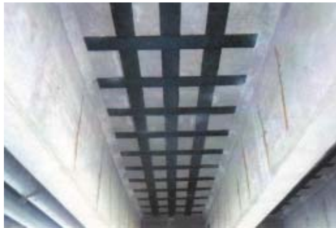
Figure 1-3: Strengthening of Concrete Bridge Deck
