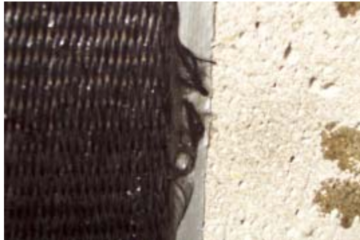
Figure 3-15: Fiber Placement over Duct Tape
