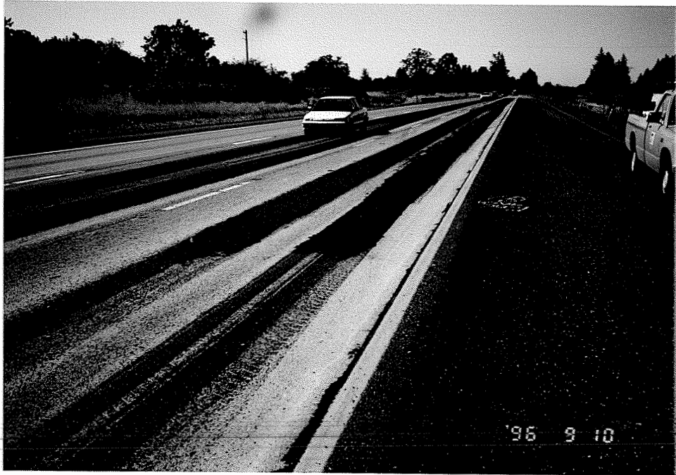
Figure 3.1 Leveling course on center and left lane.
