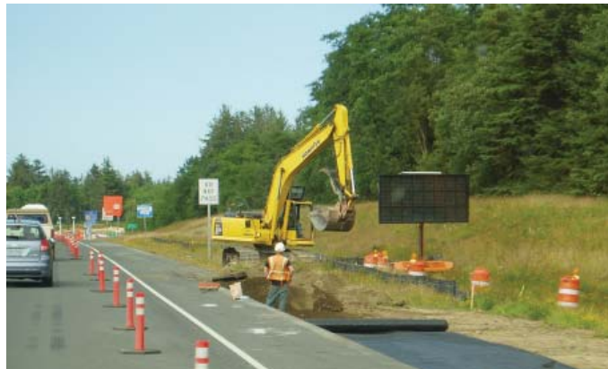
Workers on the US 101 - Youngs Bay bridge project
