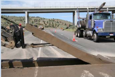
Excavation of travel lane for moisture investigation
