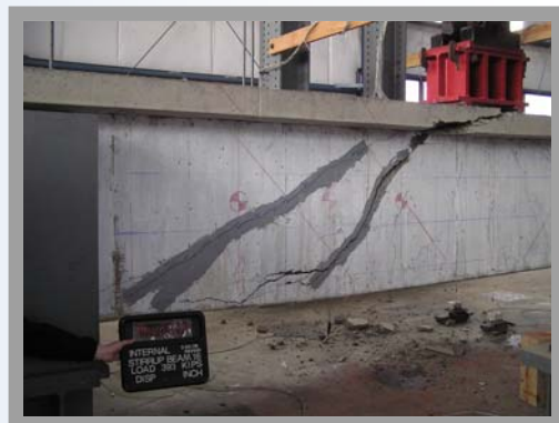
Girder after failure
