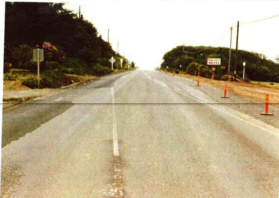
6/10/77 Southbound view from sta. 150.
