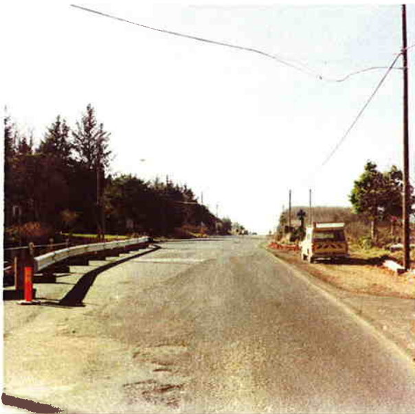
2/14/77 Looking south from 1875+50 Reflectorized buttons barely visible (weather sunny).
