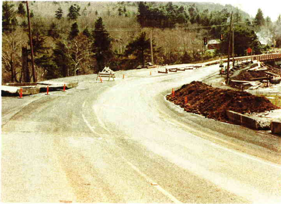
Looking southerly from station 1869+40.
