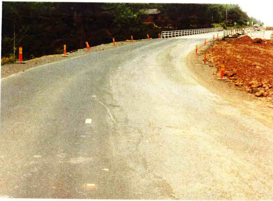
6/10/77 Southbound view from near sta. 1872. Note nailed reflector in foreground and use of reflective tape.
