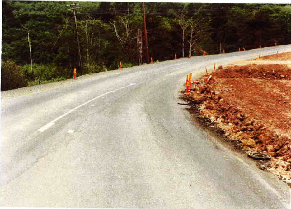
6/10/77 Southbound view from near sta. 1869.
