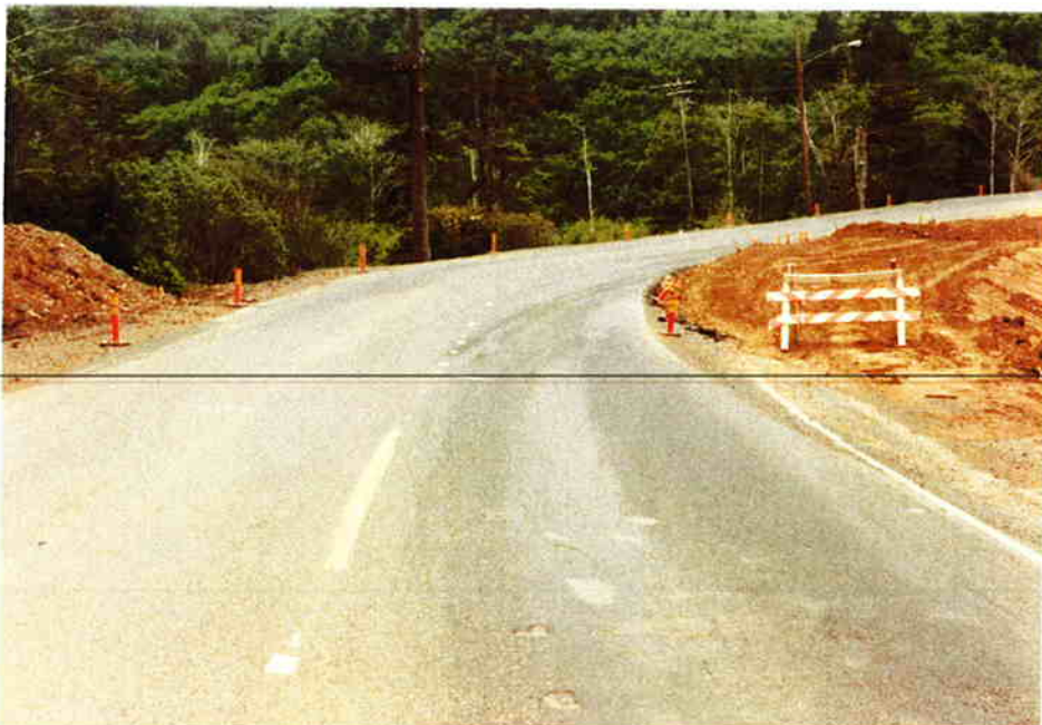
6/10/77 Southbound view from near sta. 1868.
