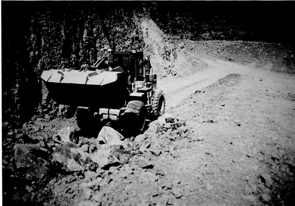
Figure 2.4: Ritchie Test Ditch
