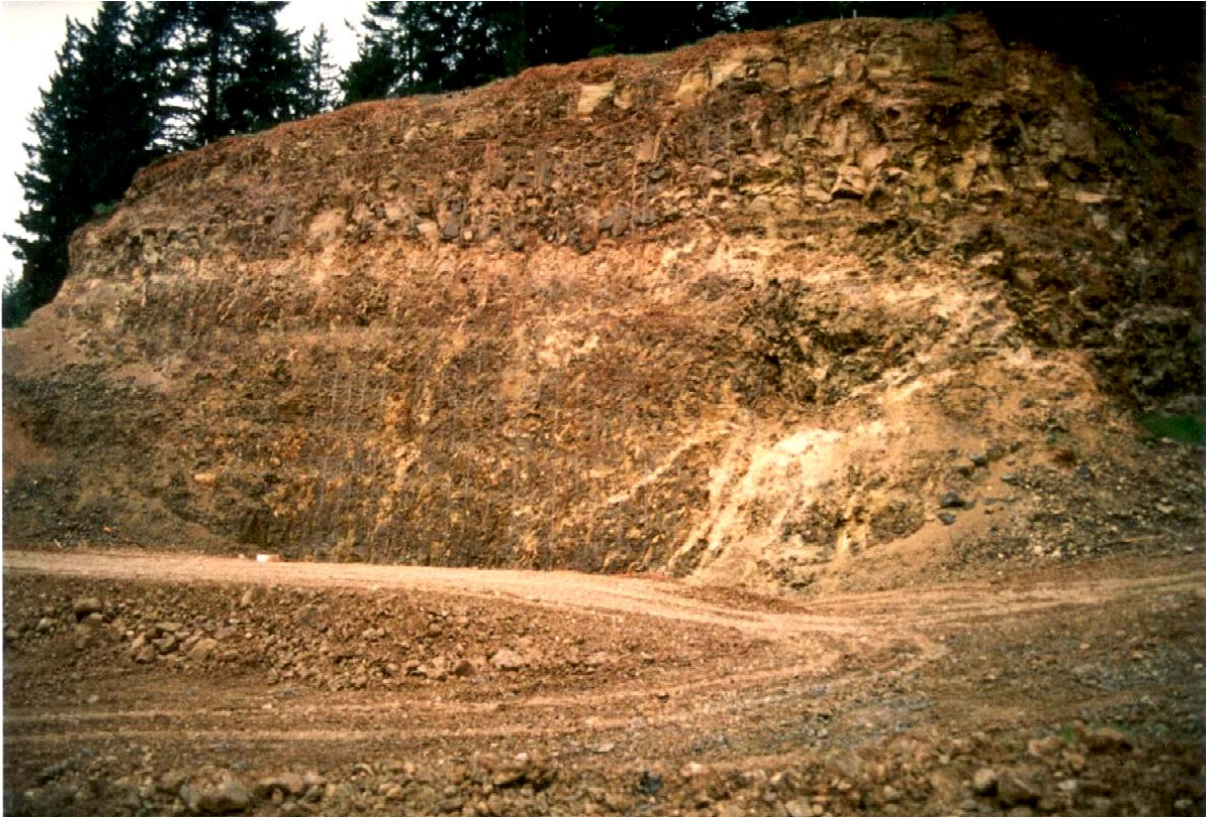
Figure 3.2: 80-foot high, 0.25H:1V presplit slope (Oregon test site)
