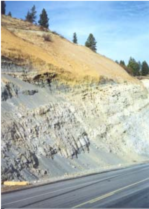
Photo 2: Looking Eastward at the cut after construction note rockfall mesh
