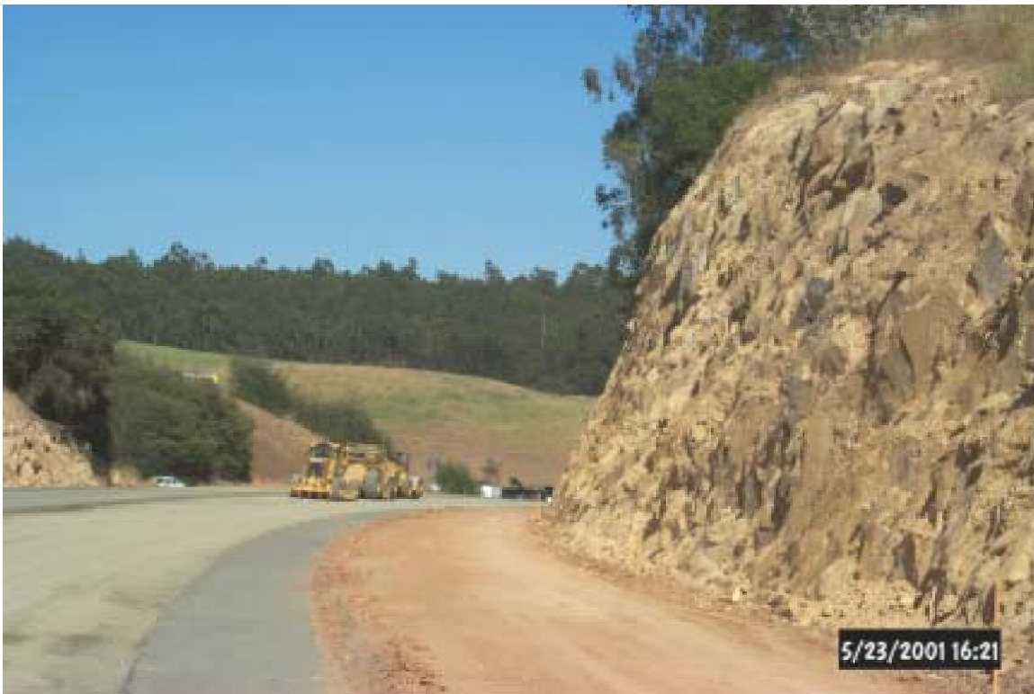
Photo 1: Cut Slope with Catchment
