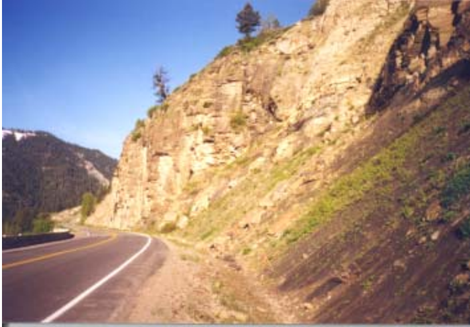
Photo 1: The cut slope looking west before construction
