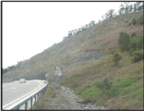
Corning By-Pass Slope: Westbound
