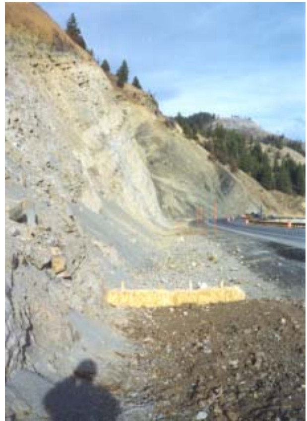
Photo 3: Looking eastward after construction note rock catchment
