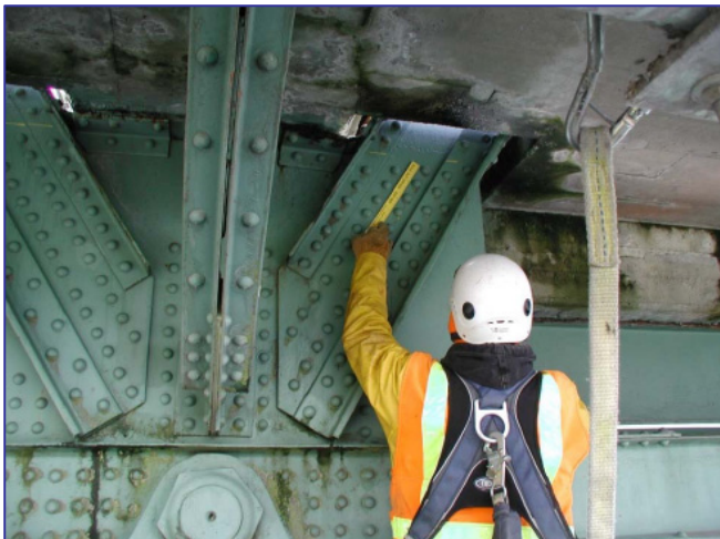
Traditional method of acquiring dimensional data for a truss connection
