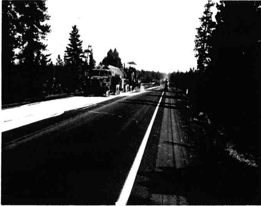
a) Overview of Lime Addition Process
