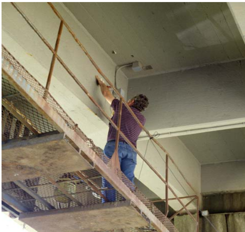
Figure 3.5: Conductive carbon paint anode CP zones on the north end of the Yaquina Bay Bridge, installed in 1986.
