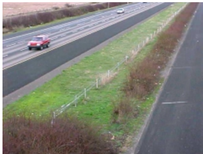
Three-cable median barrier system on I-5.
