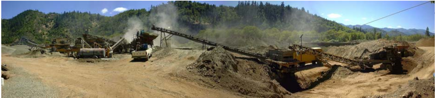
Portable Crusher Setup on Kummer Bar for I-5 Paving Job (Summer 1999)
