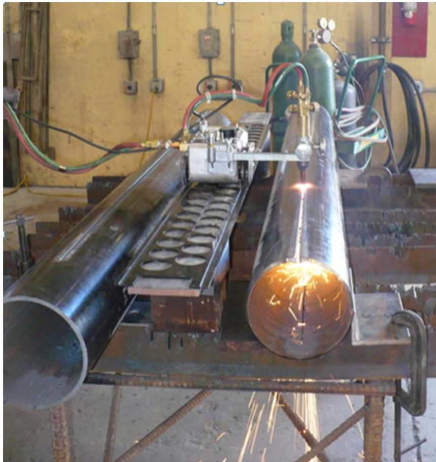
Figure 3.13: Splitting the pipe stiffener with a track torch
