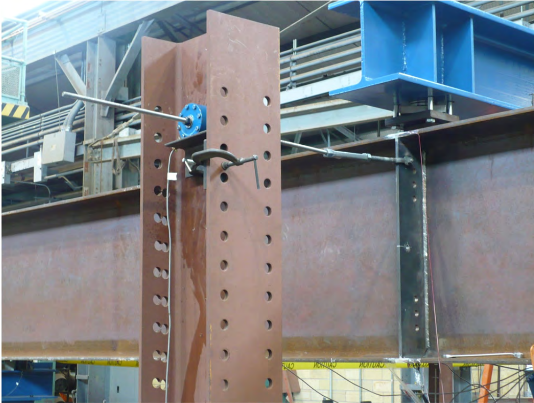
Figure 3.20: Torsional load test turnbuckle loading system
