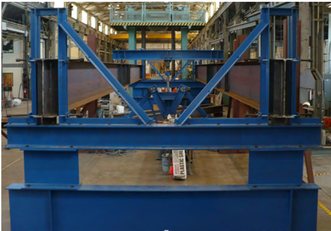
Figure 3.12: GBP1 and GBP2 in the twin girder buckling test frame (looking north)
