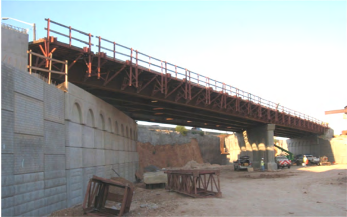
Figure 1.2: Skewed straight steel girder bridge
