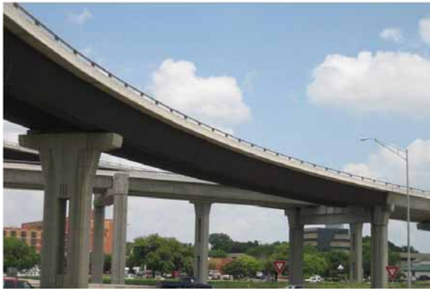
Figure 1.3: A typical two-box steel girder bridge in Austin, TX
