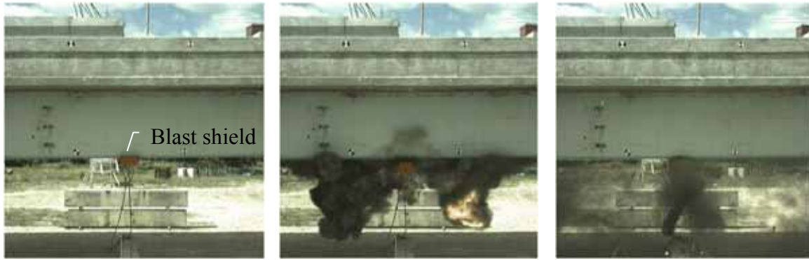
Figure 1.5: First bridge fracture test (bottom flange simulated fracture by explosion)
