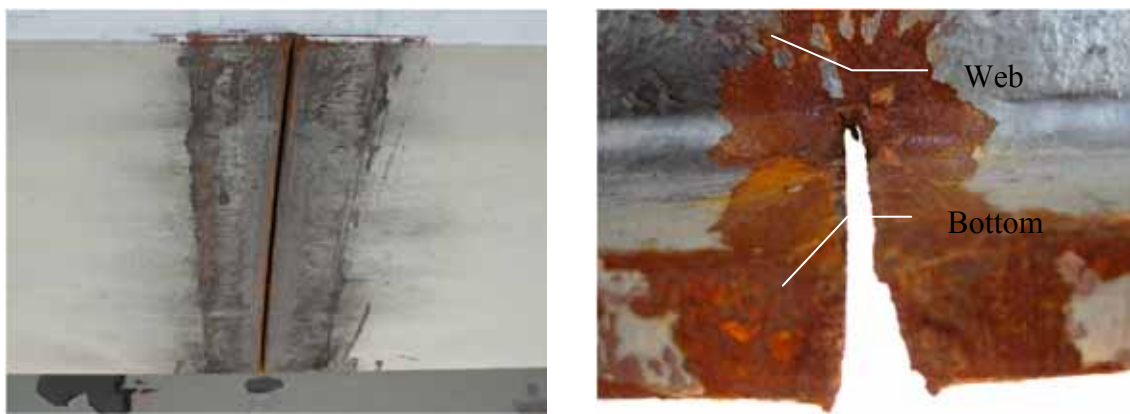
(a) Full cut of the bottom flange
