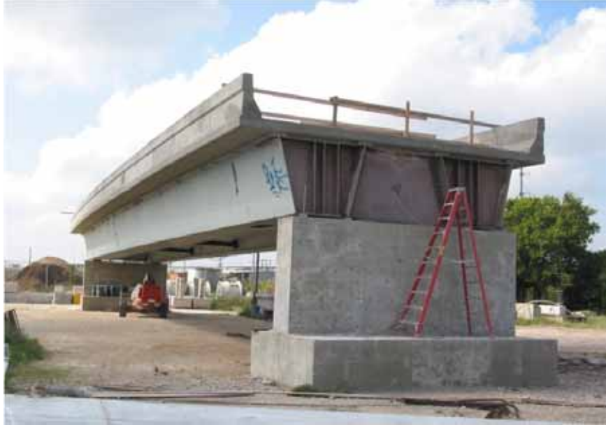
Figure 1.4: The FSEL test-bridge
