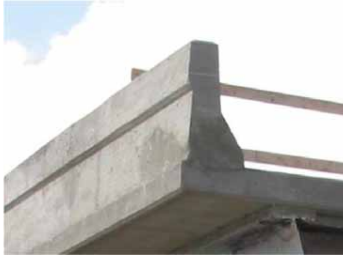
Figure 6.7: T501 rail of FSEL bridge
