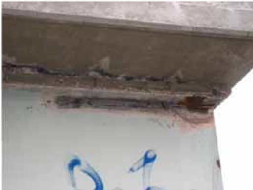
(e) Shear and tension failure of shear studs along FG-Out haunch
