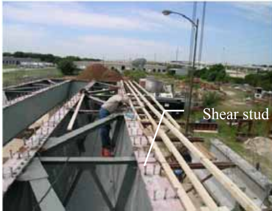
(a) Shear studs installed on top flange
