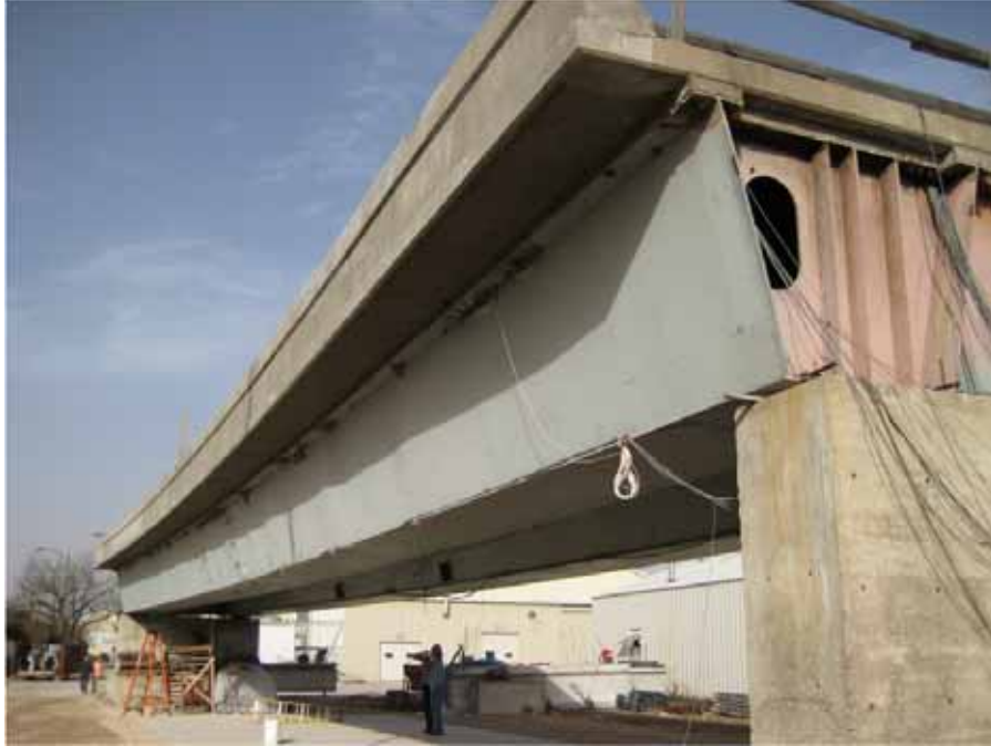
Figure 5.1: Full-scale test bridge
