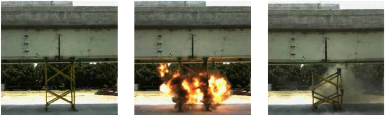
Figure 5.10: Second bridge fracture test (bottom flange and web removal)
