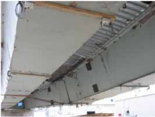
(b) Haunch separation along FG-In haunch
