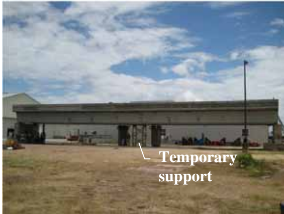
(a) Second bridge test setup
