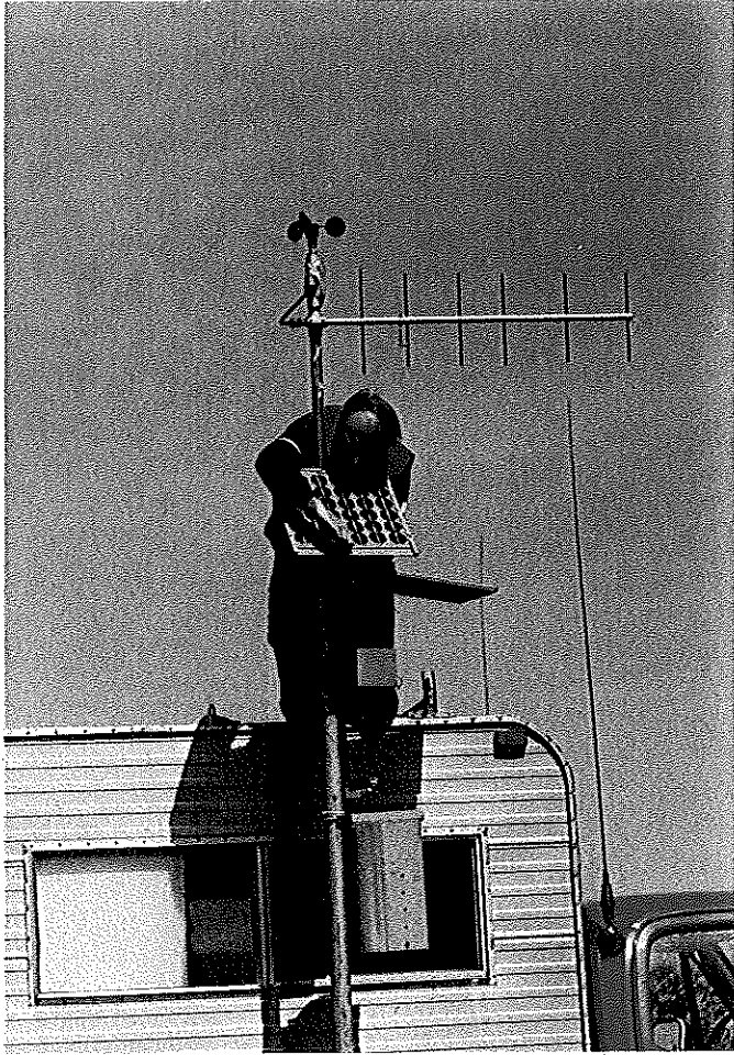
Figure 1 Installing Telemetry Station
