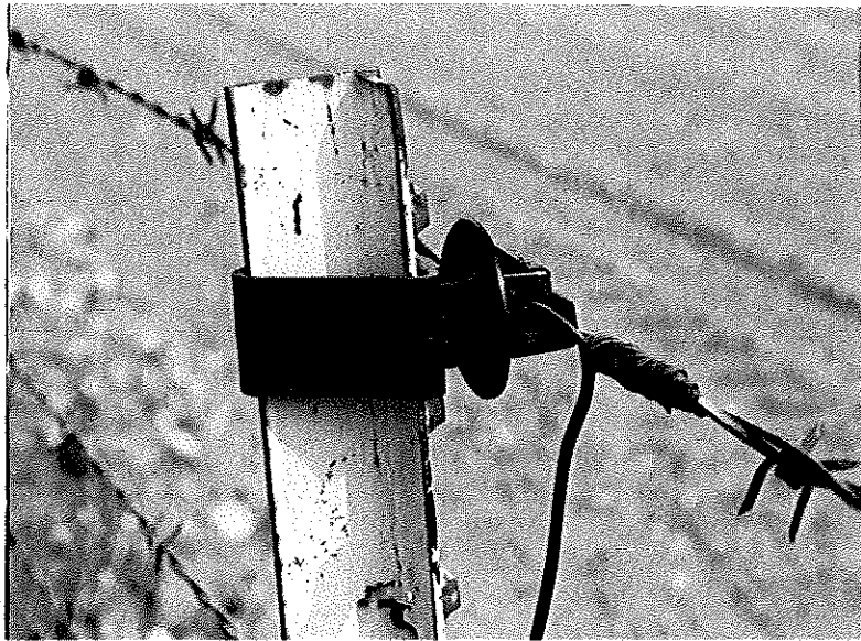
Figure 13. Fence Insulator
