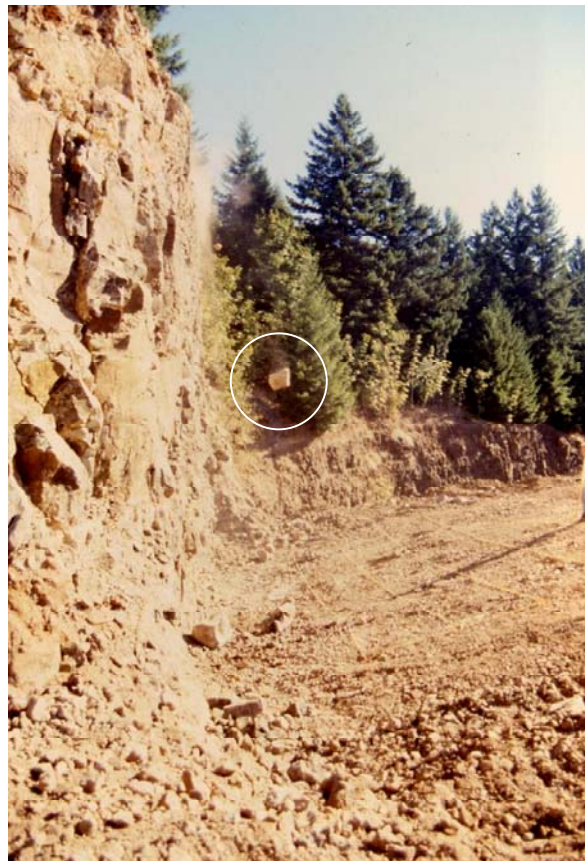
Rockfall testing; 40-foot high vertical presplit slope. Circle denotes test rock. Grid lines (middle-right) are for measuring impact and roll out distances.
