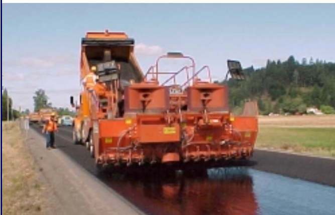
Applying Asphalt Cement Chip Seals
