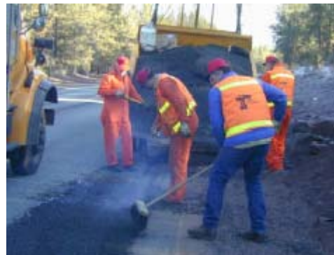
Bend maintenance crew repairs potholes
