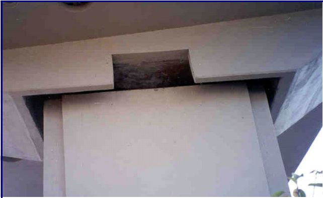
An inspection access for the base isolation bearings
