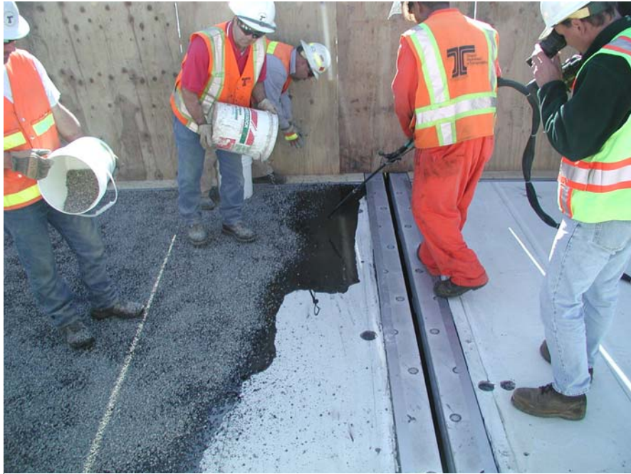
Applying wearing surface on the Siuslaw River Bridge
