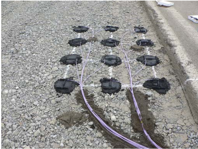
Strain gage layout over the rubbilized concrete base
