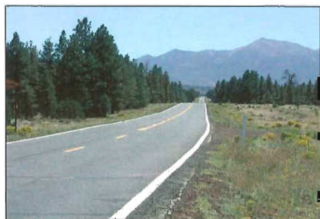
Typical view of US 180 roadway, southbound near boundary that separates Coconino and Kaibab national forests.
