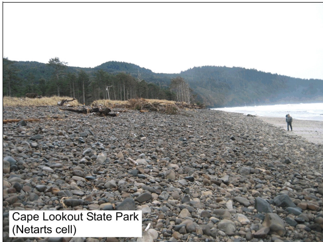
Dynamic revetment at Cape Lookout State Park near Netarts, Oregon.
